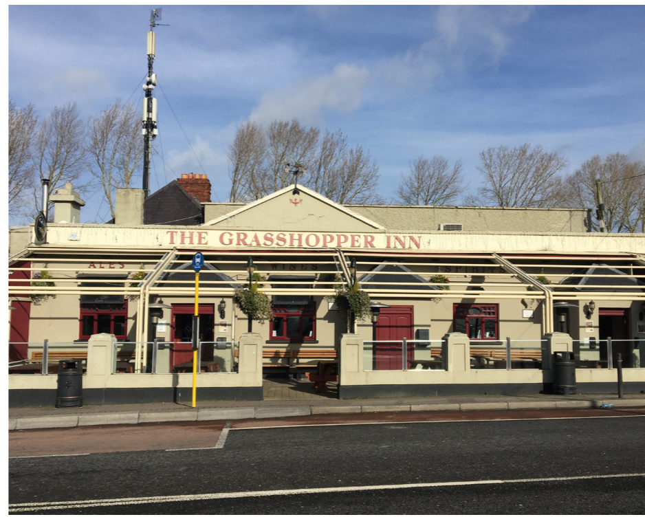
5. A surviving and vibrant community oriented pub- restaurant
