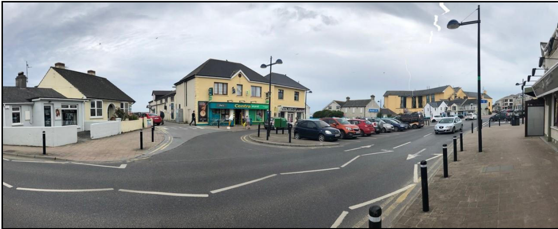
FIGURE 2.4: VIEW OF THE R150 LOOKING SOUTH TOWARDS THE PUBLIC CAR PARK
