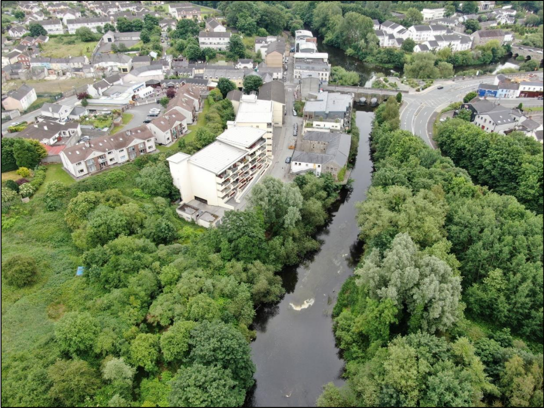
Figure 19: Apartments at Southern end of Flowerhill
