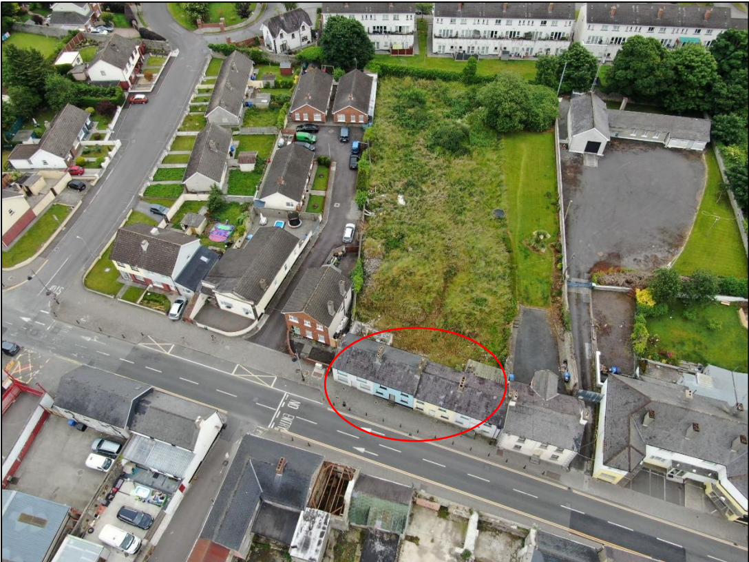
Figure 21: Example of derelict buildings on Flowerhill
