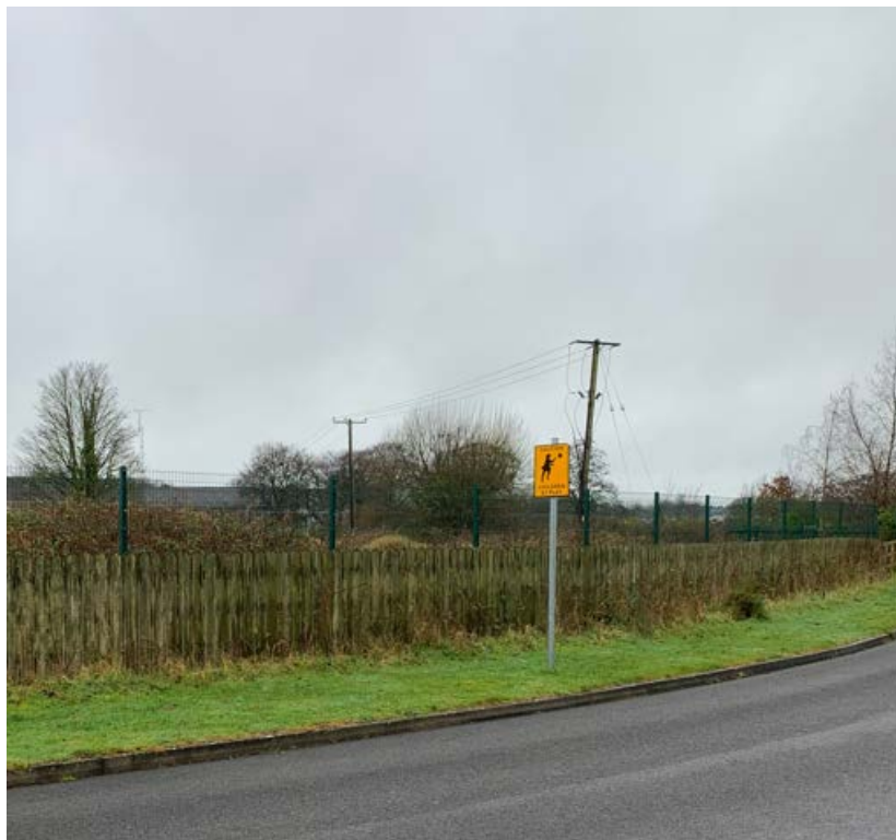
Plate 2-11: Existing Warning Sign
