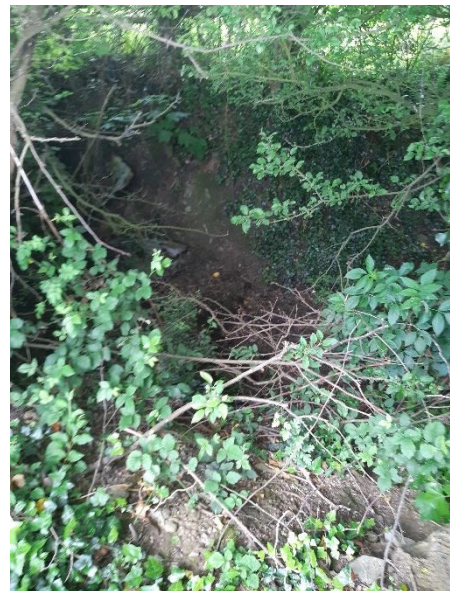
Dry Ditch Along Western Boundary
