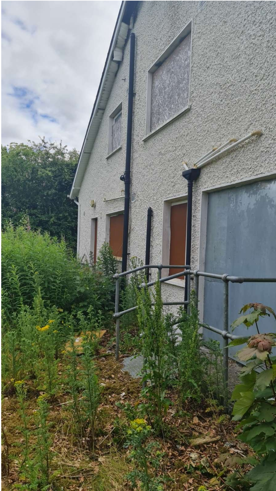
Close up of rear elevation, with all opes boarded up.
