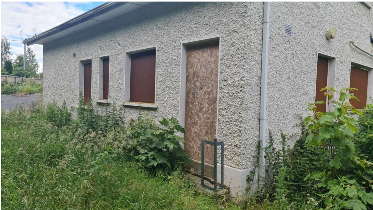
Side elevation with all opes boarded up.
