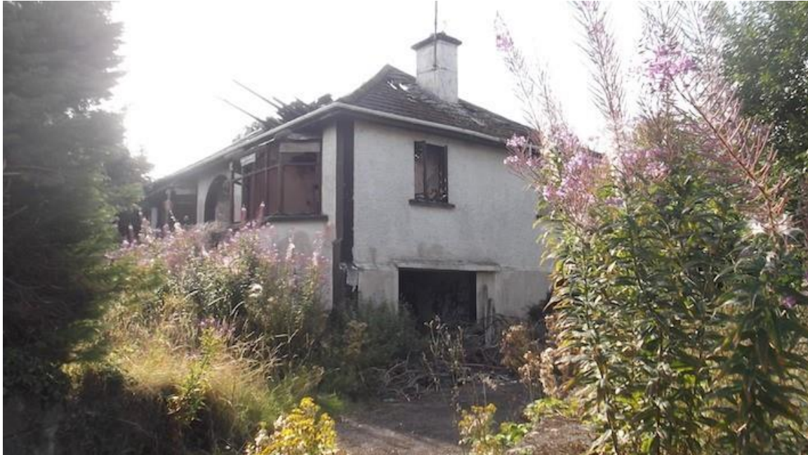
Fig. 1. Area proposed for development is almost entirely built-up (BL3).
