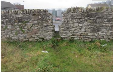
Western Boundary / Railway Yard Pedestrian stile facing W
