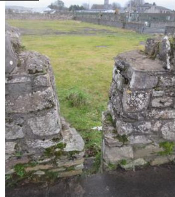
Western Boundary / Railway Yard Pedestrian stile facing E
