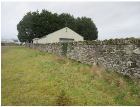
Eastern boundary wall. Southern end
