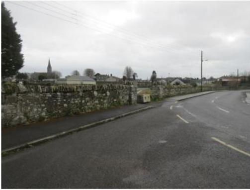
N end. Modern gate. Facing S
