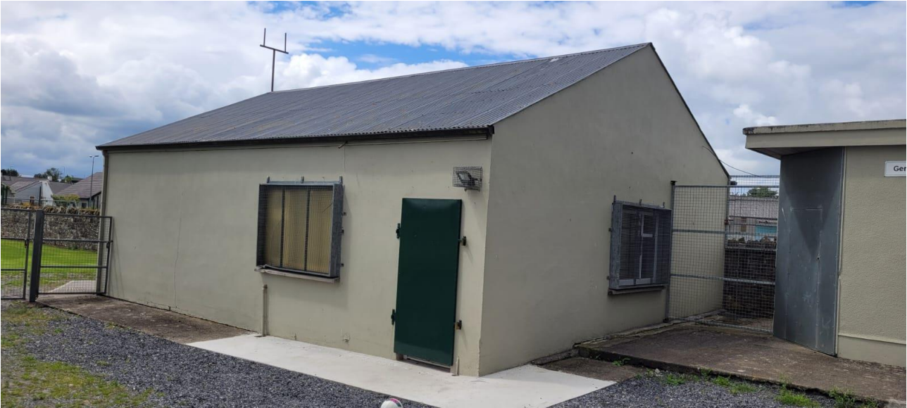
Plate 2: A-roof single storey structure immediately adjacent to proposed development area.
