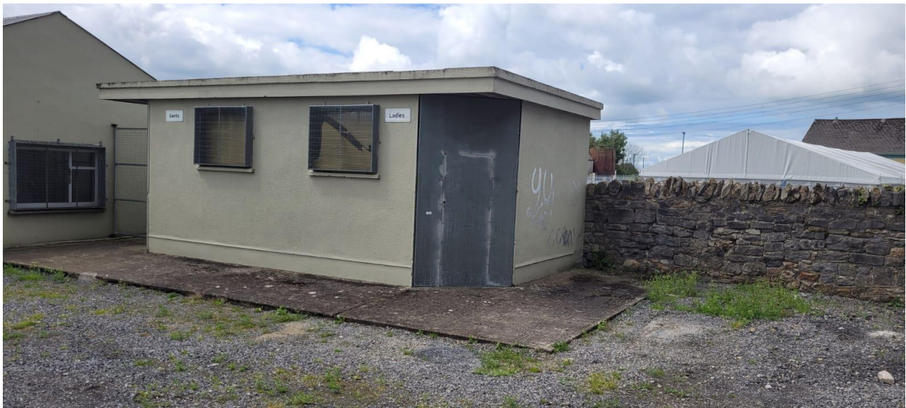
Plate1: Toilet block immediately adjacent to proposed development area.
