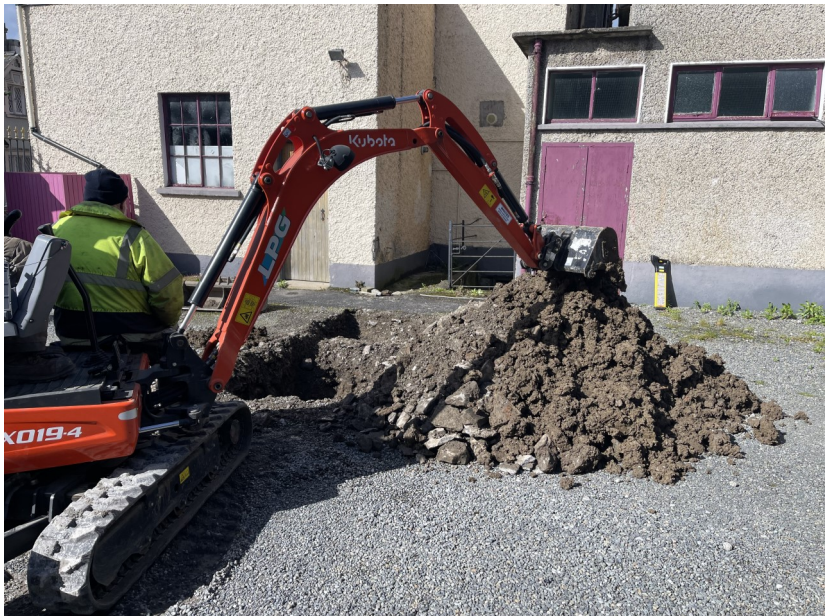
Plate 11: Location of Trench 4, south of Market House, looking northwest.
