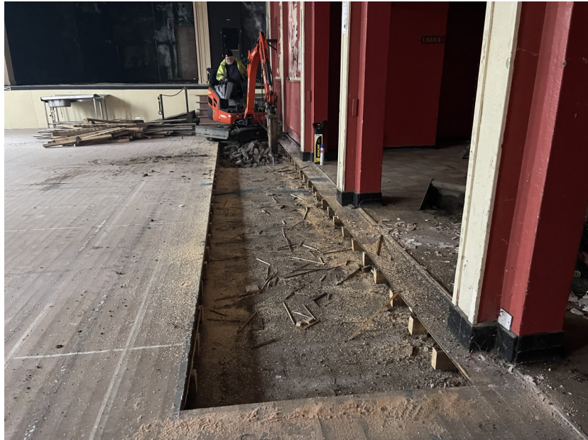
Plate 5: Location of Trench 1 inside ballroom, looking southeast.
