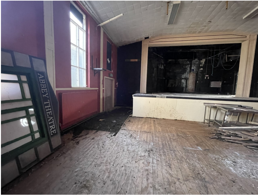
Plate 9: Location of Trench 3 inside ballroom, looking southeast.
