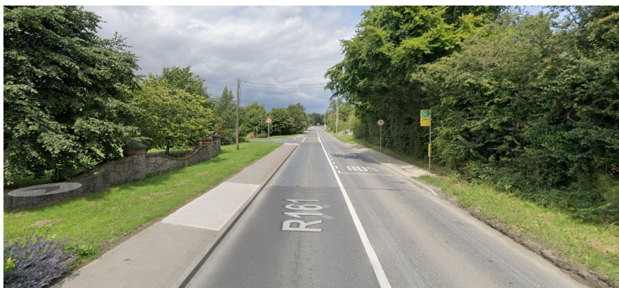
Figure 3a: Before - South of Canterbrook Estate on the R161 Road
