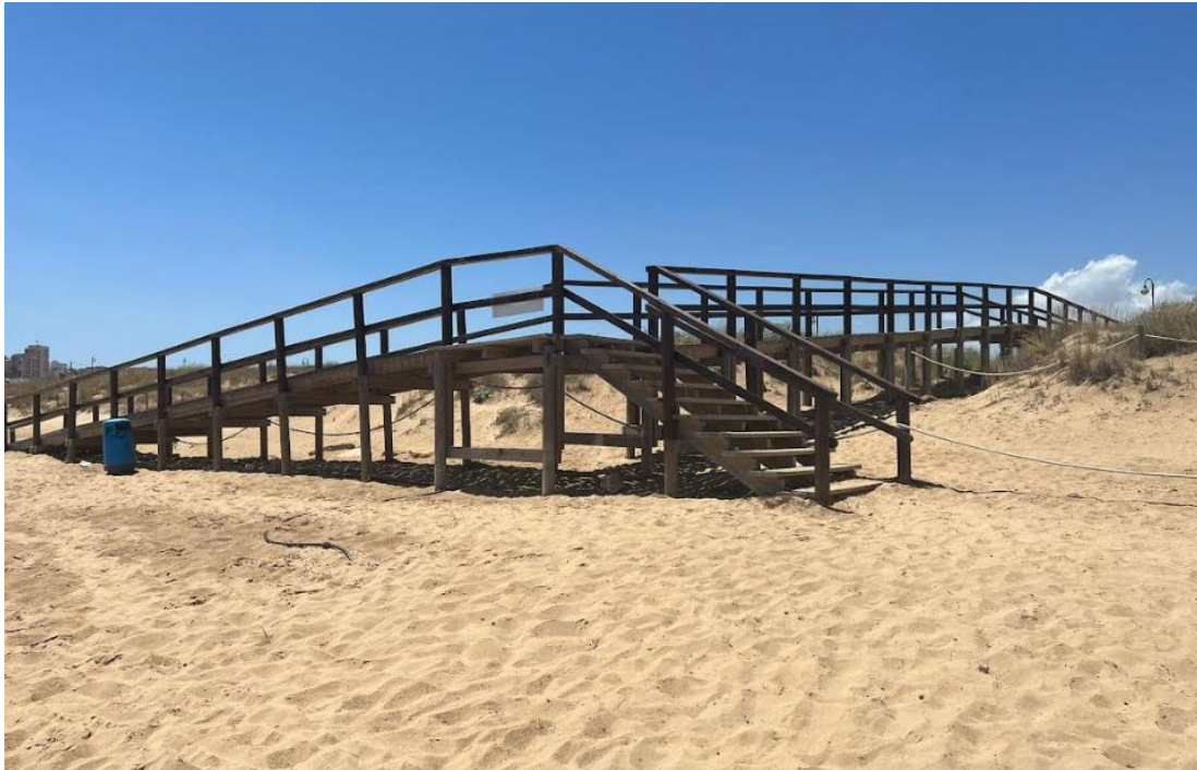
Photo 2: An example of a raised Boardwalk (Credit Sharon Tolan)
