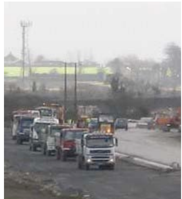
M4 corridor under construction.
