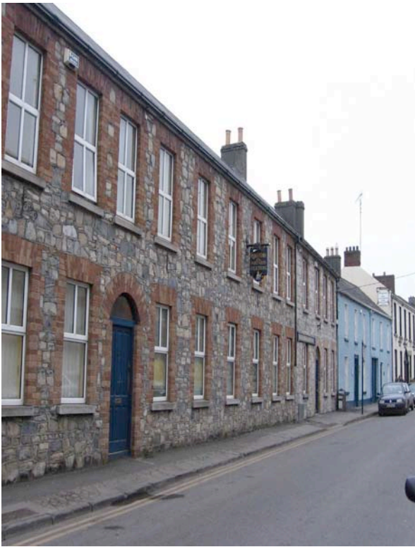
Restoration of historic buildings, Trim
