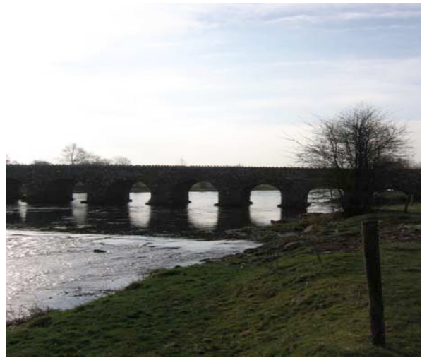
Bridge over River Boyne near Bective Abbey
