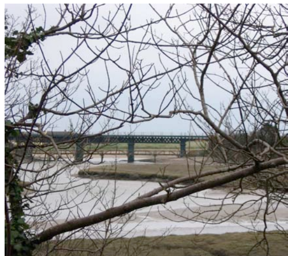
Railway bridge over the Nanny estuary near Laytown
