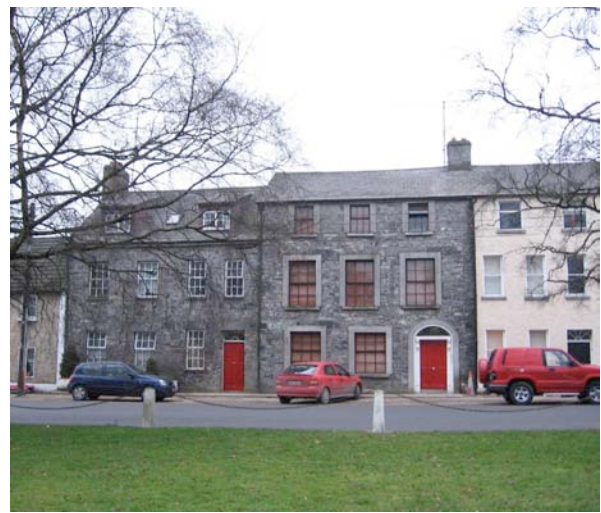
Period houses in the estate village of Summerhill.
