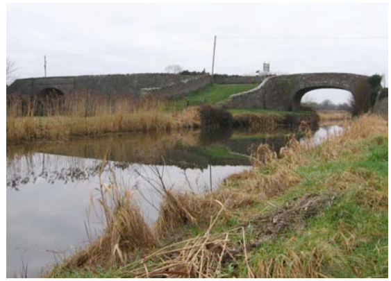
Canal bridge over Royal Canal outside Enfield.
