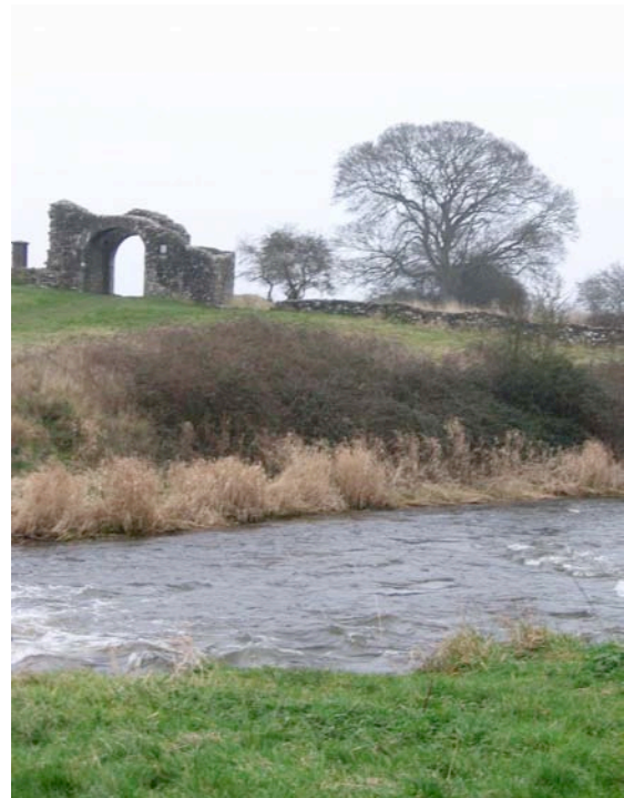
Trim town walls
