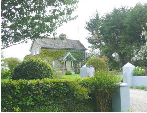
STOREY AND HALF COTTAGE
