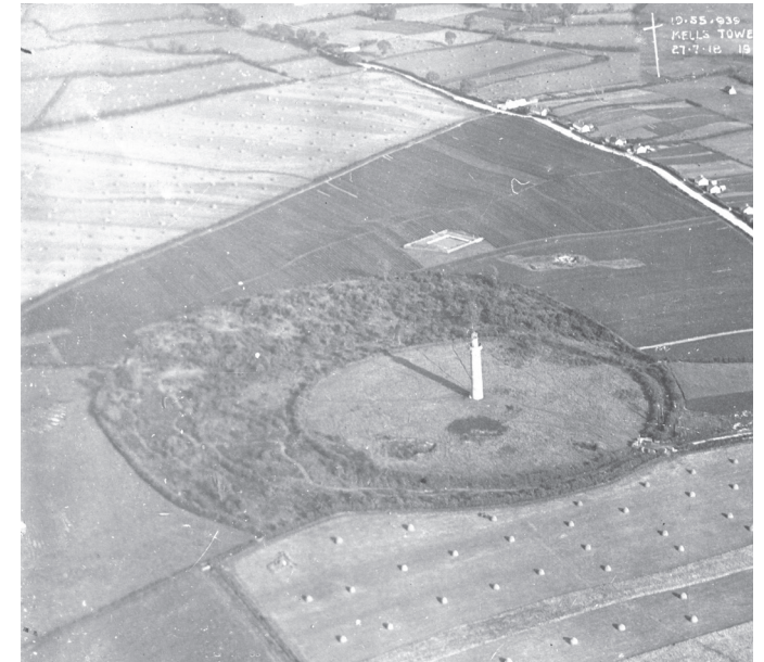
Figure 2.11: Aerial view of the Tower of Lloyd taken by RAF Bi-plane in 1918 | South Dublin Libraries, Dimmock Collection
