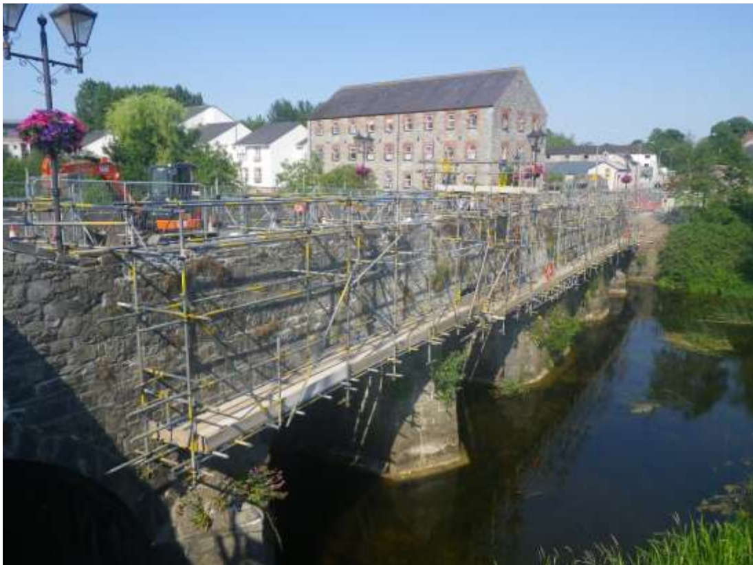
Plate 2.1: Boardwalk construction along New Bridge
