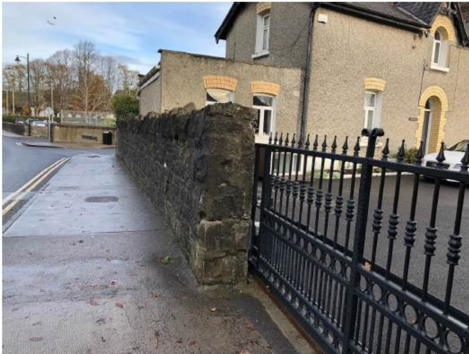
View along boundary wall to Station Master's House.
