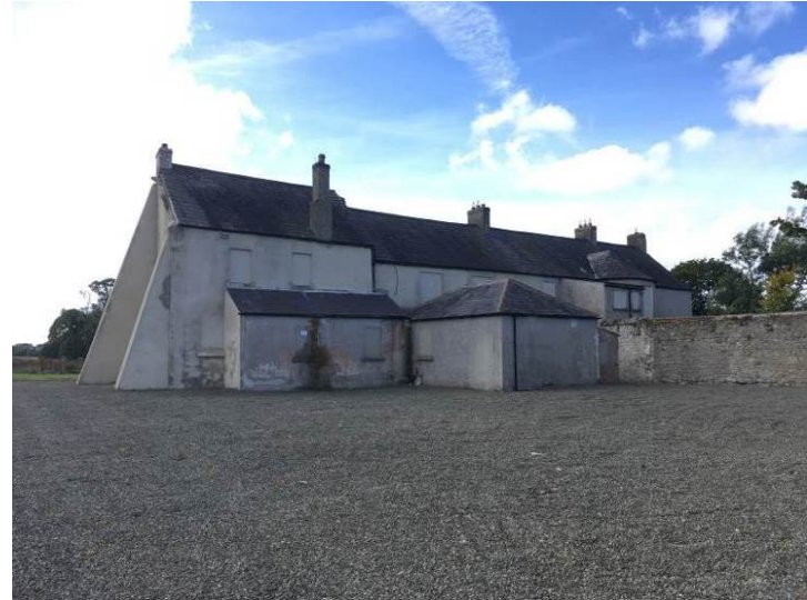
Plate 30: Violet Hill house (RPS NT025-138) following removal of convent structures, facing southwest
