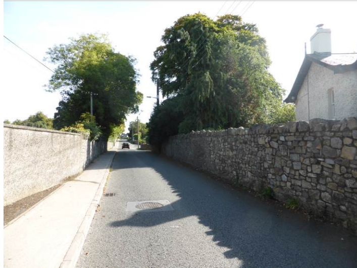
Plate 17: Boyne Cottage (NT025-133), right of shot and boundary wall, facing southeast
