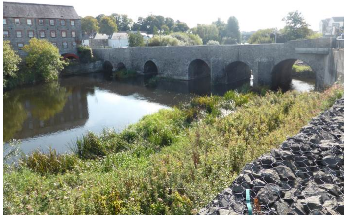
Plate 15: New Bridge (RPS NT025-115), facing southeast
