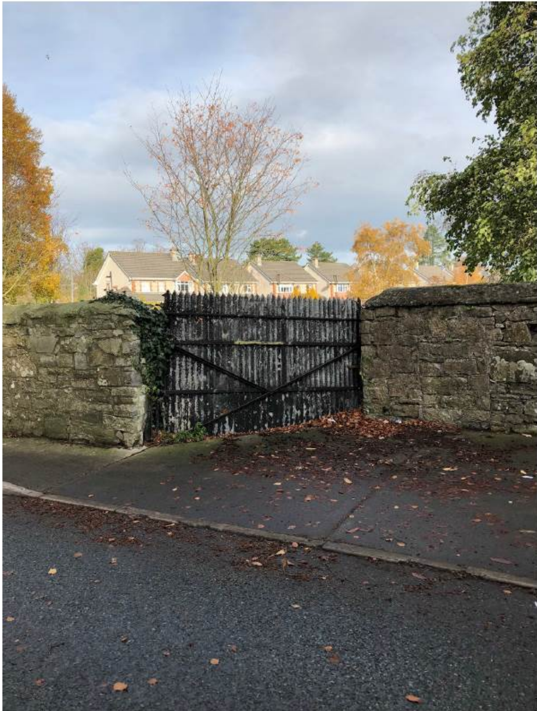
Detail of gap in wall close to castle, the end of proposed wall realignment on the north side of the road.
