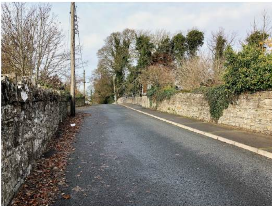
View of incline towards bridge, with cock and hen walling to churchyard on south side of road. Note overhead services along the road.
