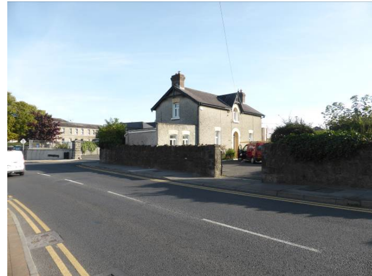
Plate 8: Station Master's House (RPS NT025-156), facing northeast
