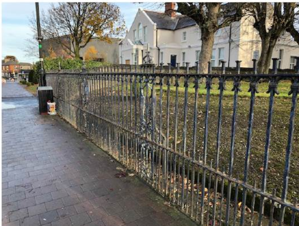
View along railings showing extent of corrosion and low base.
