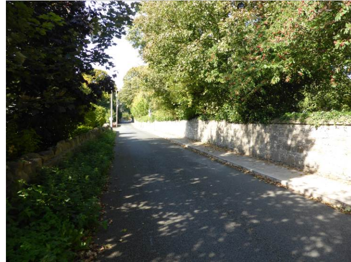
Plate 18: Demesne wall associated with Athlumney House (NT025-131), facing west-northwest
