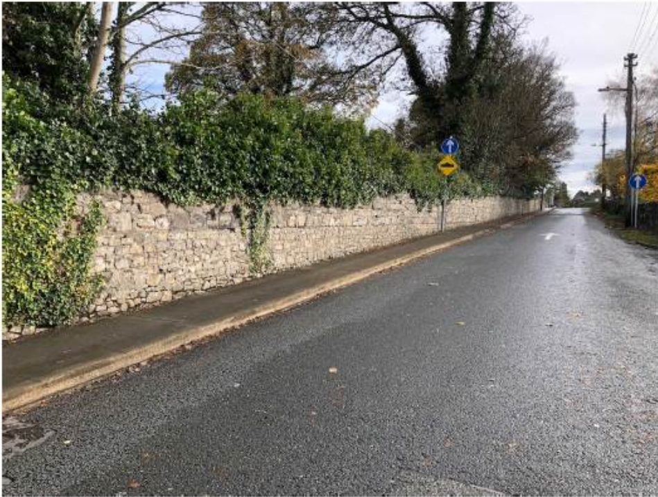
View looking east along Loreto Convent wall showing coursed rubble laid in horizontal bands, possible on top of eighteenth century wall below.
