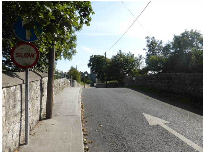
Plate 19: View southeast over railway bridge (RPS NT025-135)
