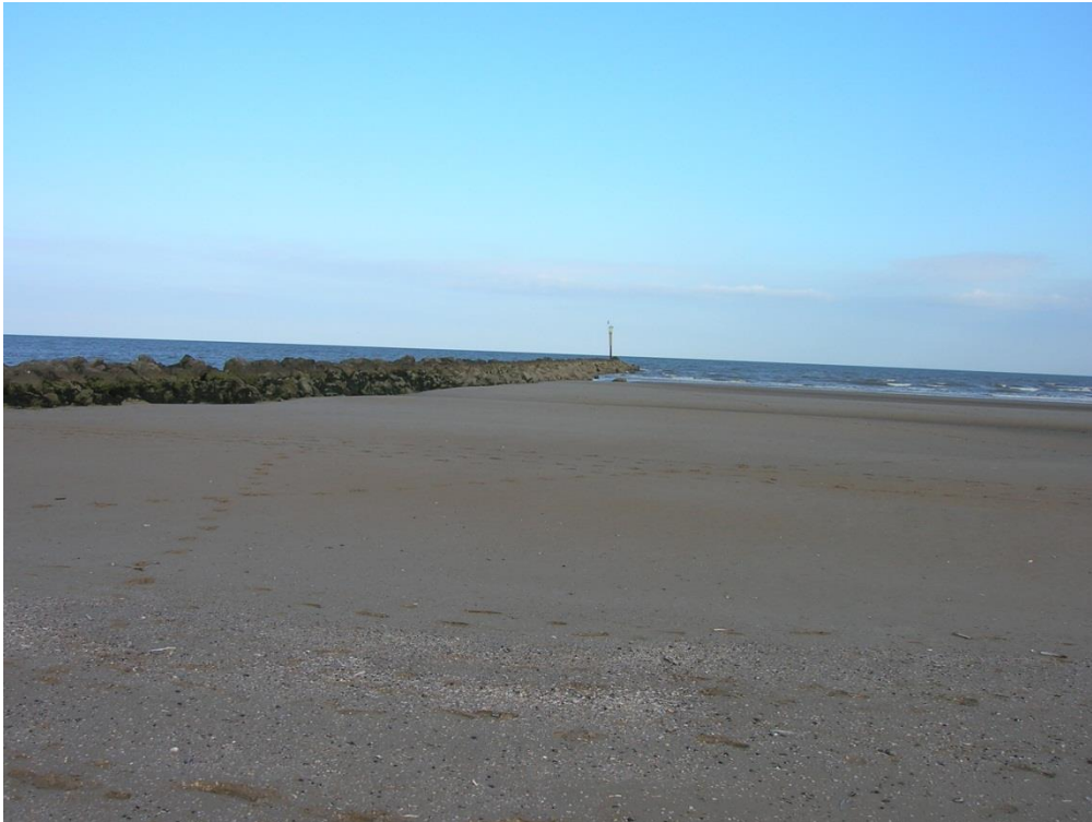
Photograph 7.7: View of deposited sand extending out towards seaward end of training walls
