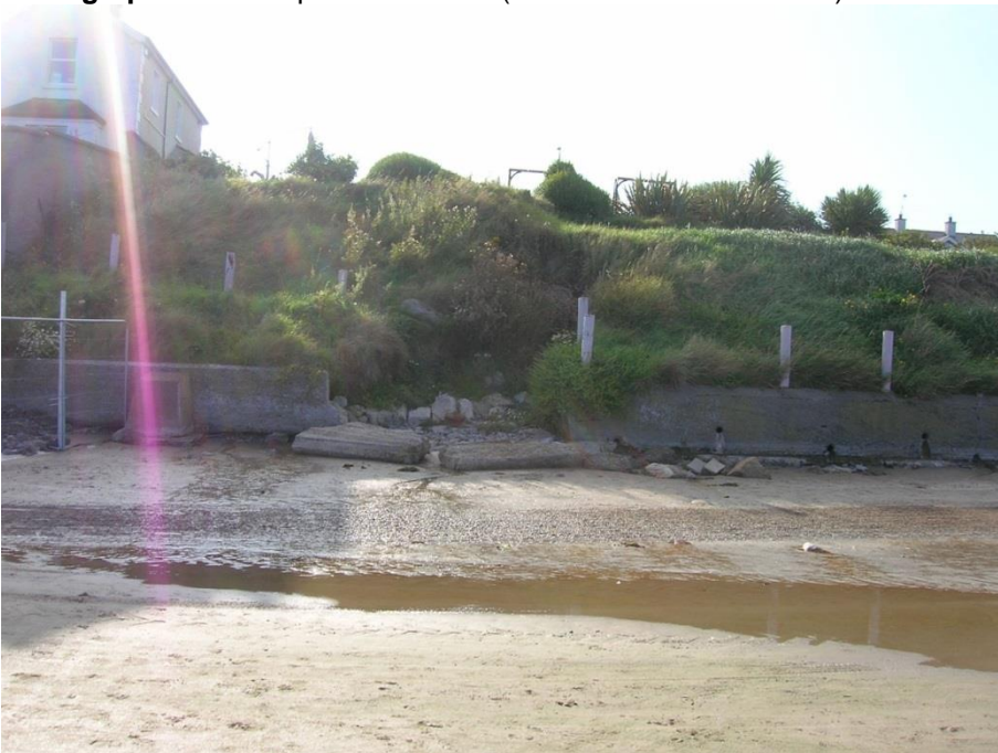
Photograph 7.3: Collapse of sea wall (note wet sand conditions)
