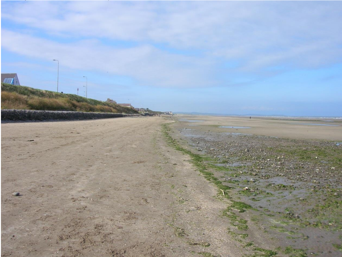
Photograph 7.1: View of Laytown Beach looking north (Note Gabion Stone Cages, limited extent of upper beach and exposed stone basement)
