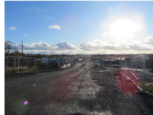
Northern Section of RORR in Construction
