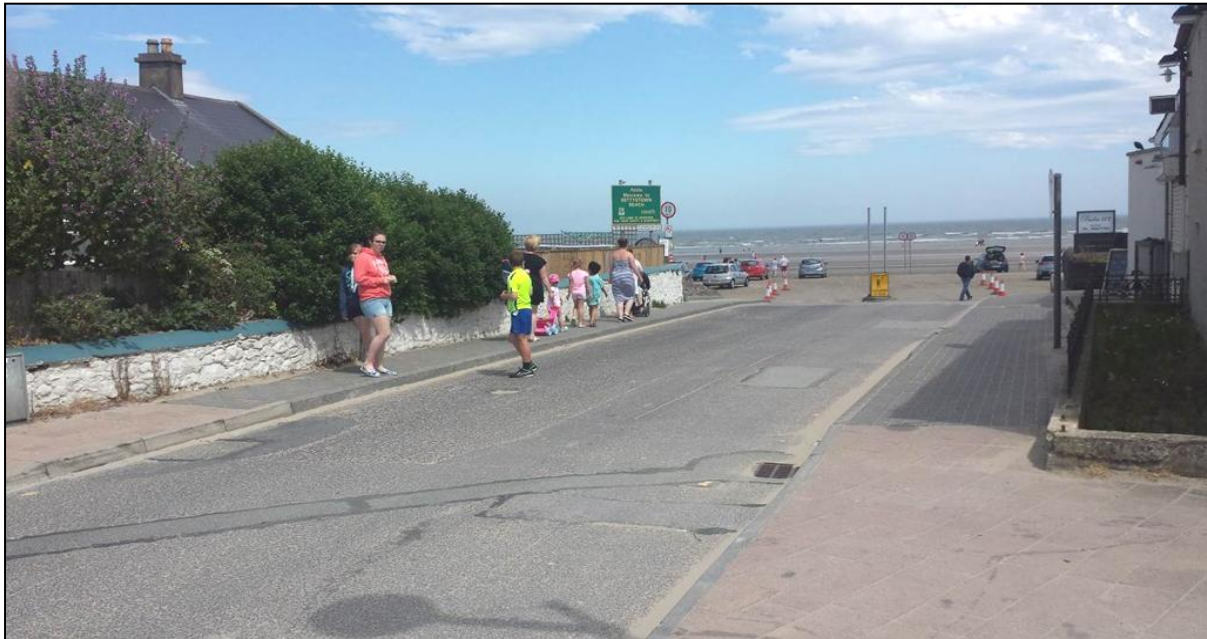
Figure 5.2: Existing Beach Access at Seaview Terrace
