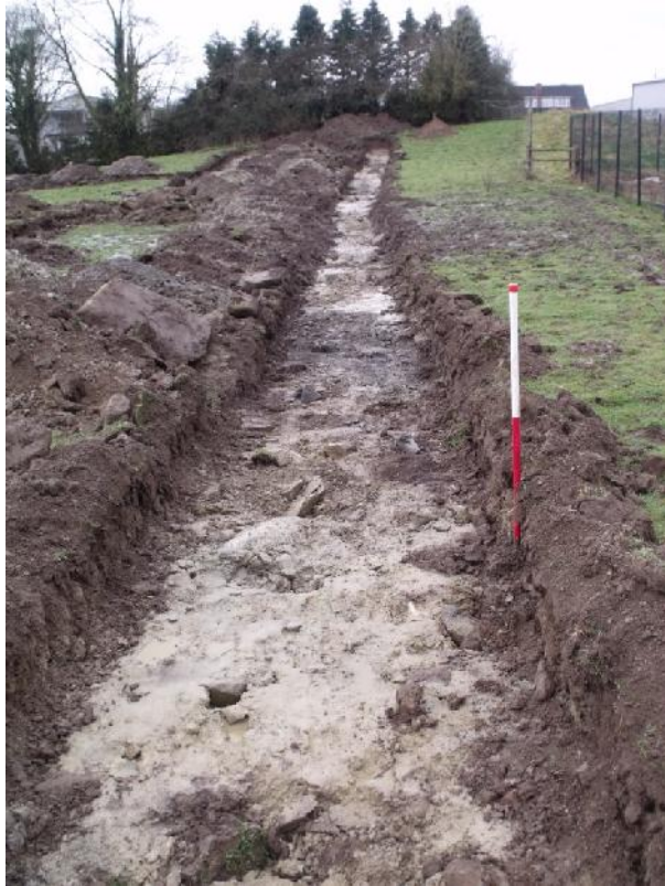
Plate 5: View of trench 7 looking W. Scale = 1 m.
