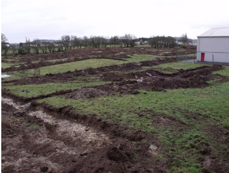
Plate 15: Overview of test trench array. Taken from NW corner of site.
