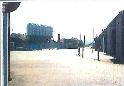
24 Cloughan St. viewed from pedestrian link to Stoney Rd.
