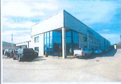
30 Kelletts Oldcastle bedding factory.
