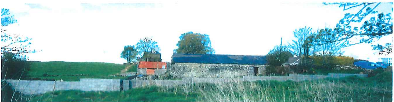
View 5 North towards existing buildings on the Stoney Road
