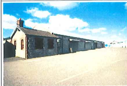
35 Oldcastle Co-Op (formerly railway station sheds).
