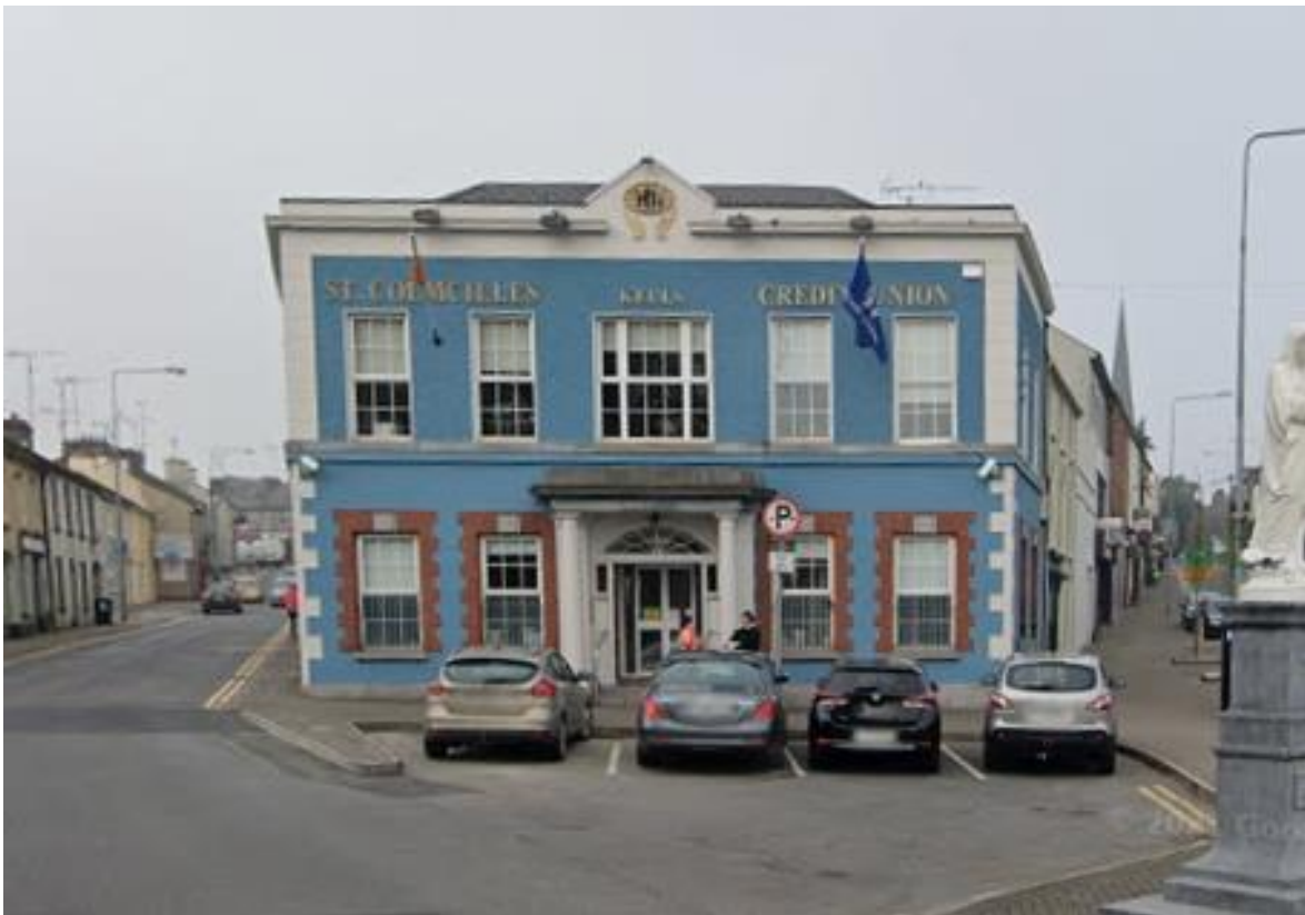
The setting of the Protected Structure is not enhanced by the car parking immediately in front of the main elevation.
