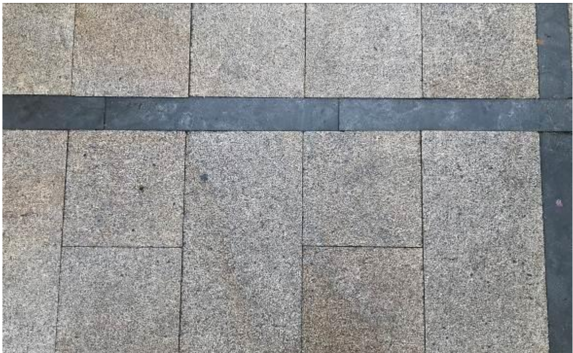
Sample of the more suitable limestone paving employed in recently completed works in Kells.
