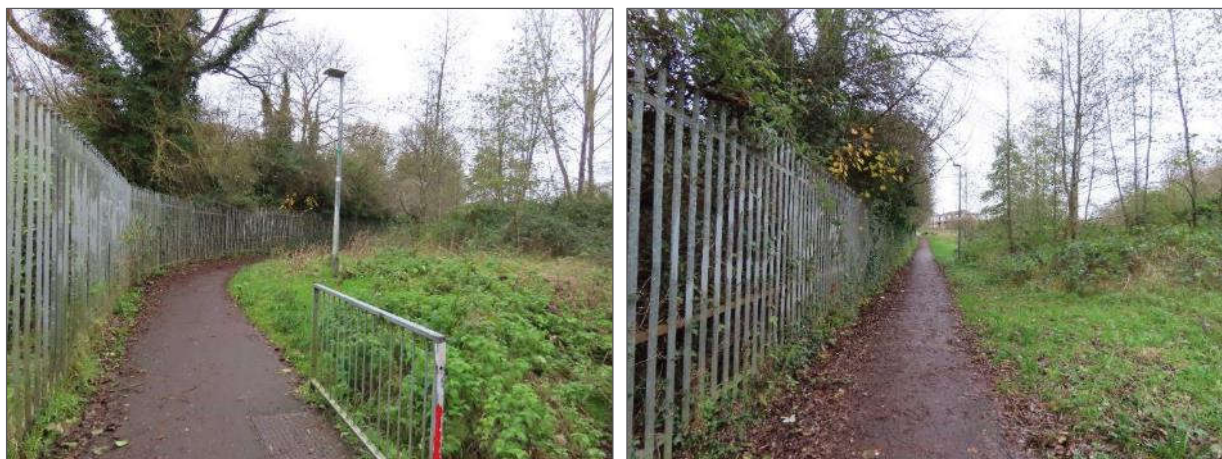
Plate 4.13 Existing path along Section 2 – immediately north of Bridge 1.
