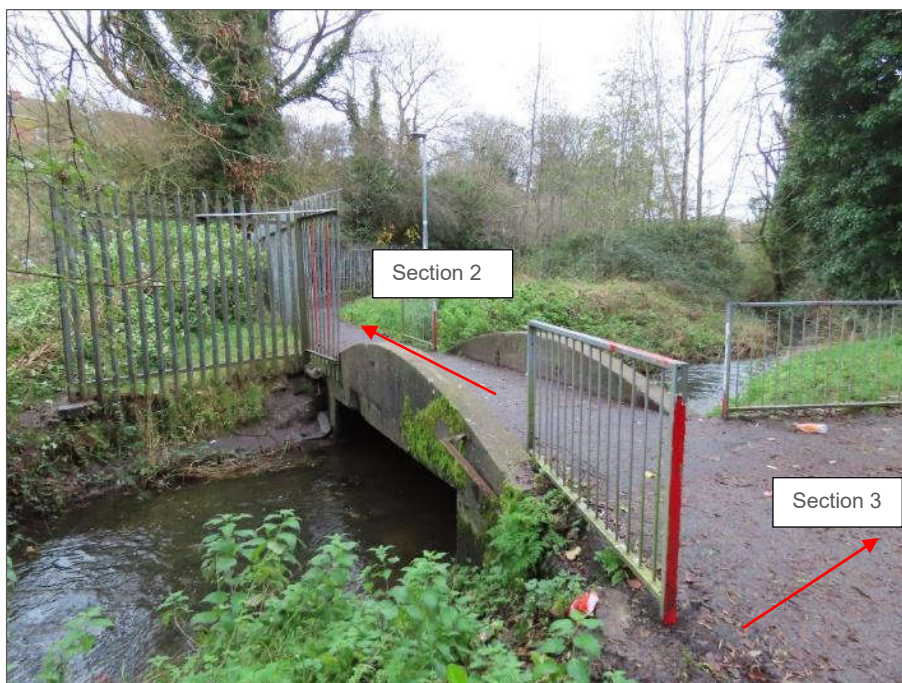
Plate 4.9 Bridge 1 – concrete culvert spanning Broadmeadow River.
