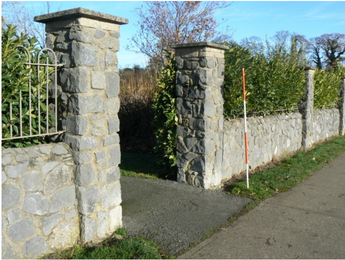
815D; Gates to The Avenue. Facing N. P1200405
