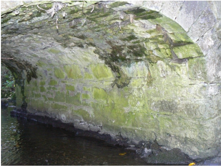
815B. Soffit under arch. P1200413
