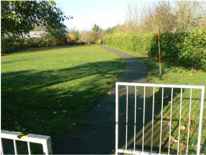
815D. Existing landscaped footpath. Facing NW. P1200407
