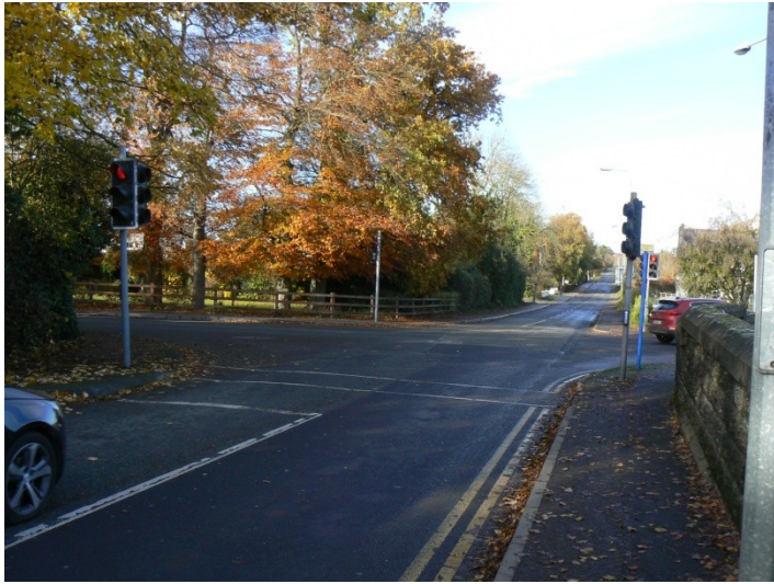
808B. Skryne Road with graveyard wall on right. Facing N. P1200482
