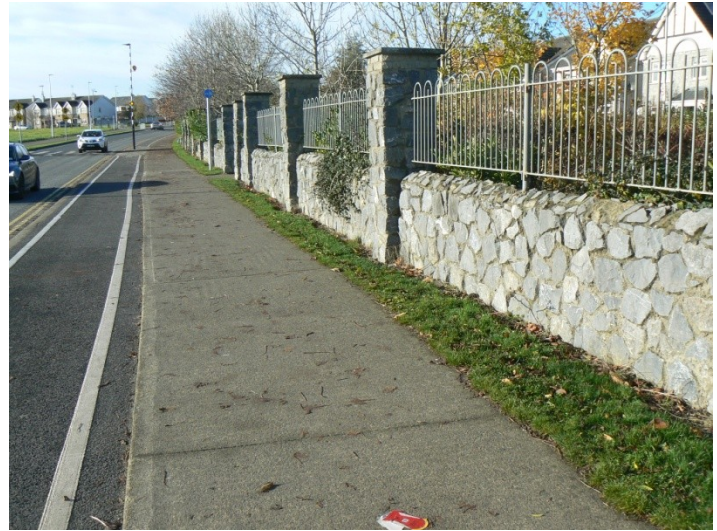
815D; Gates to The Avenue. Facing SW. P1200406
