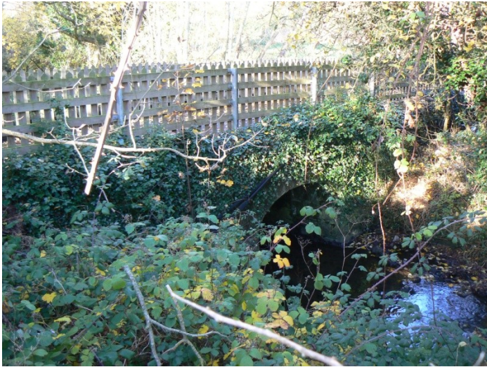
815B. Bridge E face. Facing W. P1200409
