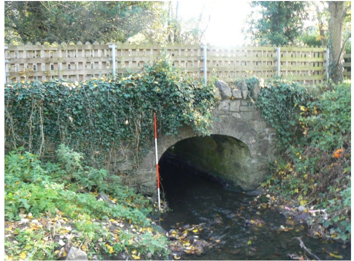
815B. Bridge W face. Facing E. P1200414
