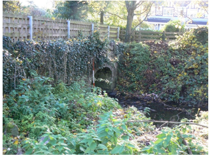
815B. Bridge W face. Facing SE. P1200416
