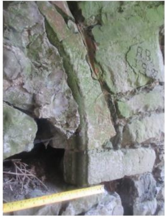
IMG_0100 'Smithy' W door S side moulding
