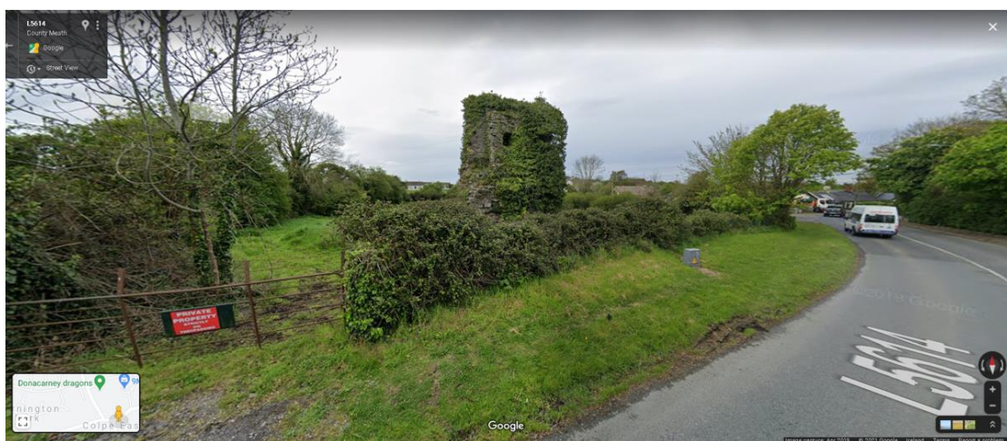
Remains of Donacarne Little Tower House ME021-009
