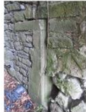
IMG_0092. N side of W door
