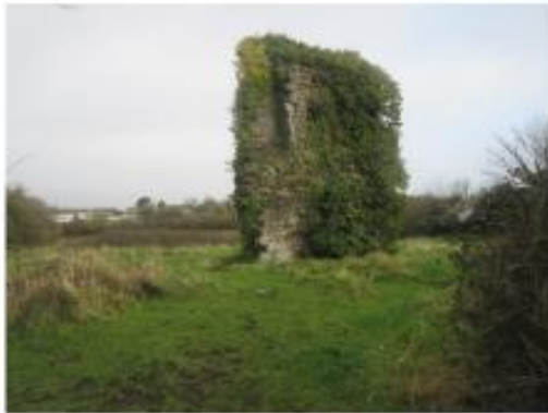
IMG_0089. Tower House ME021-009
