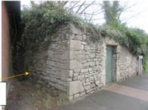
IMG_0091. Smithy W and S walls. Facing NE
