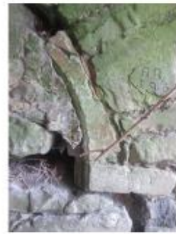
IMG_0094. Springer and arch on S side of W door
