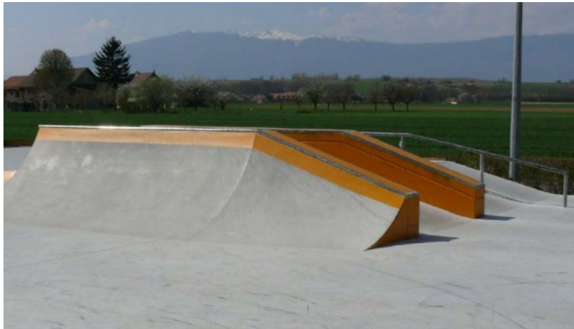
Figure 2-3 Typical Concrete Features of a Plaza Style Skate Park (Photos Source: X-Move 2 )
