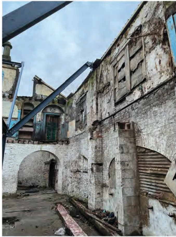
1.2 View along Western wall.jpg
