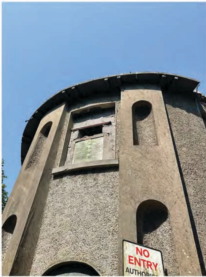
2.6 View of South buttresses.jpg
