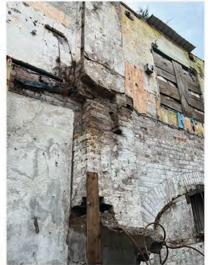
1.12 Buttress detail - East.jpg
