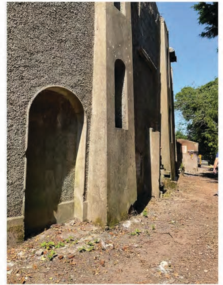
2.8 View looking North West.jpg
