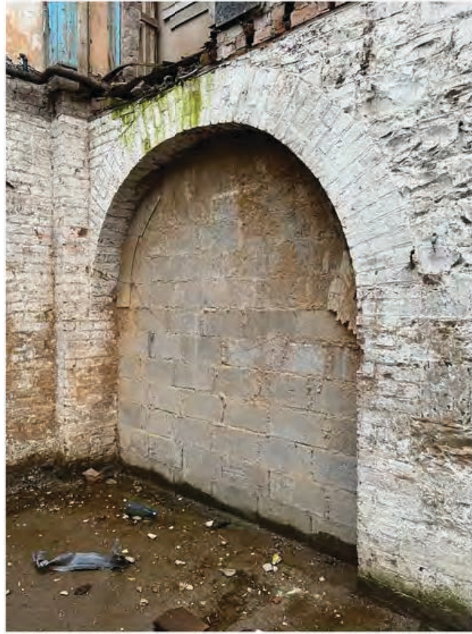
1.8 Infilled North Arch.jpg
