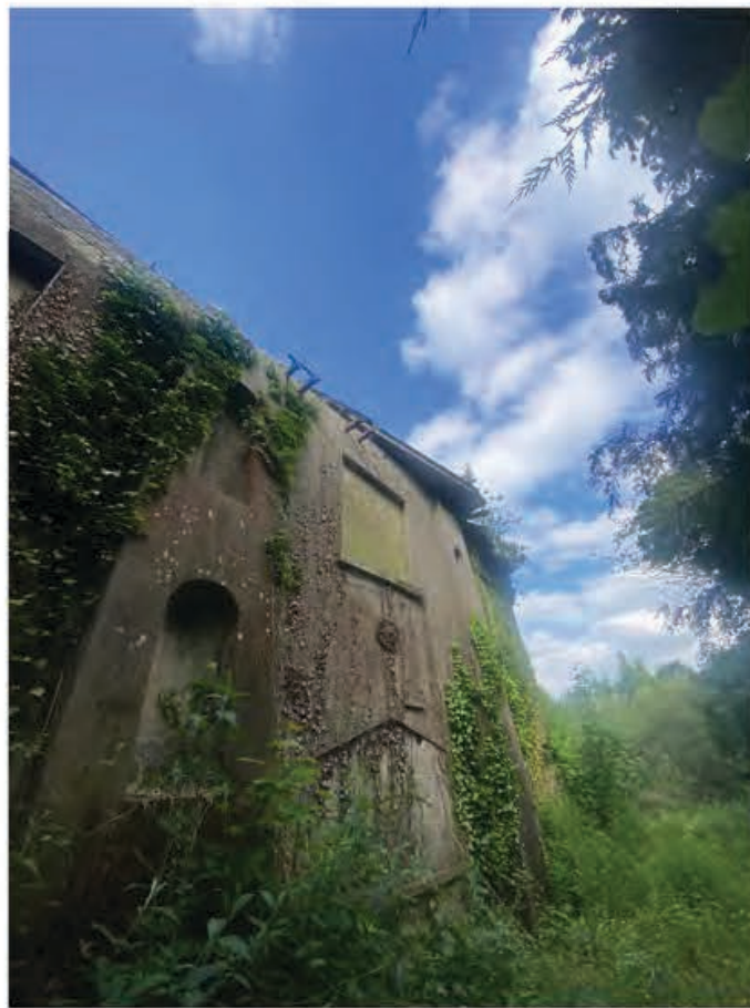
2.10 View looking South East.JPEG
