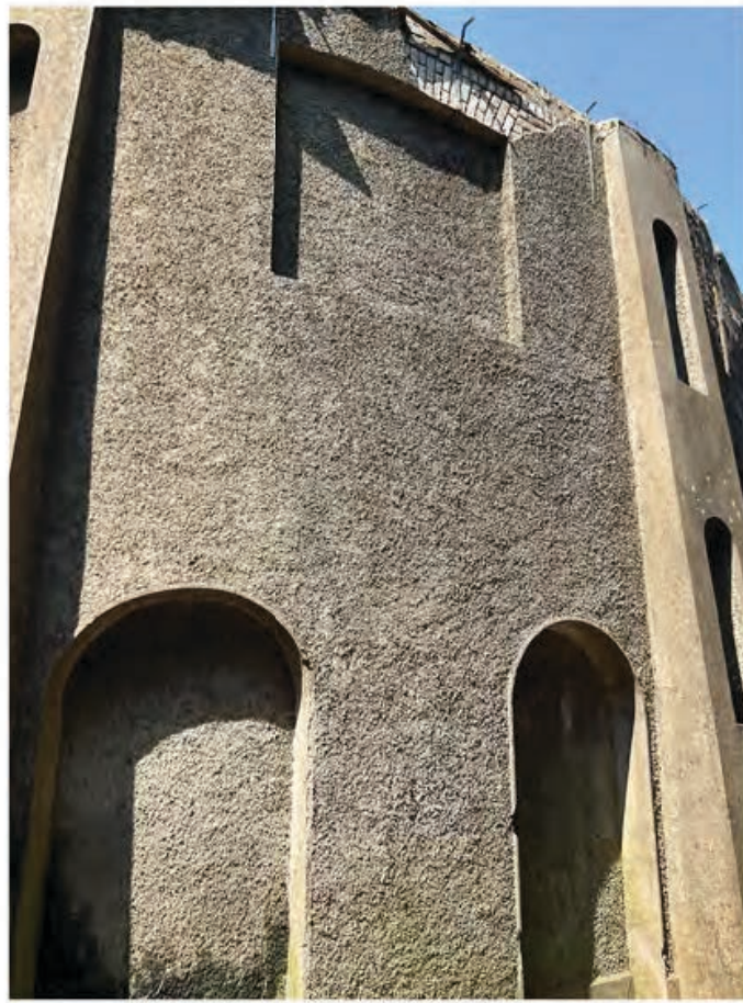
2.7 View looking North West.jpg
