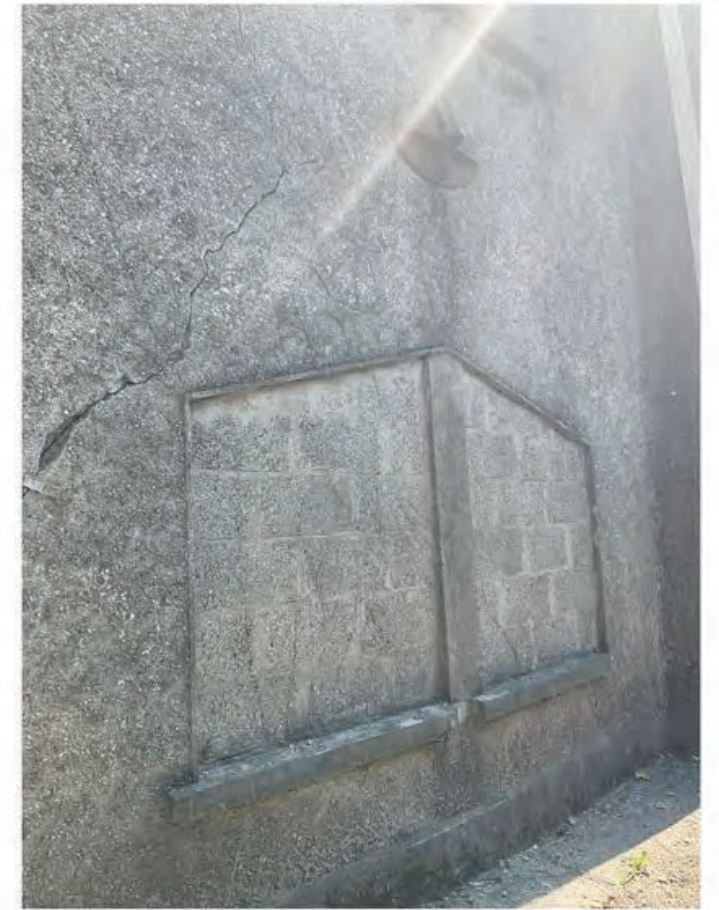
2.2 Infilled window - North West.jpg
