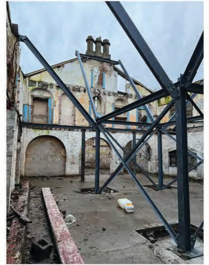
1.3 View looking North West.jpg
