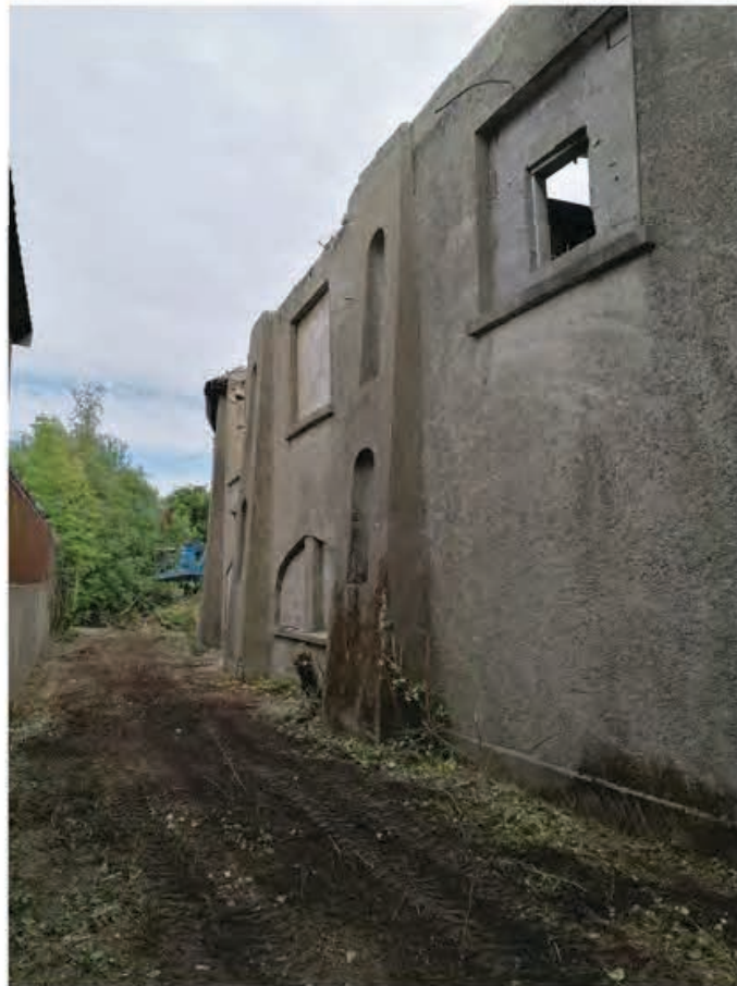
2.4 View looking North West.jpeg
