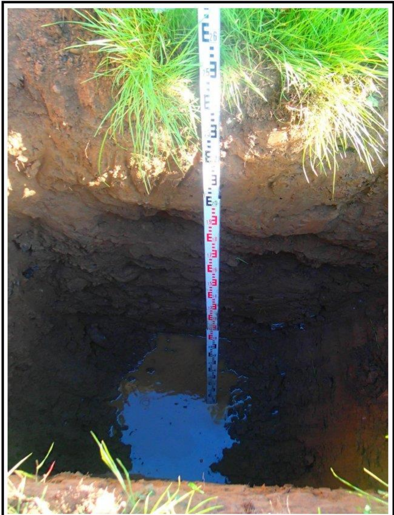
Plate A1: Profile of well drained topsoil overlying unmoistened very silty gravelly SAND with occasional cobbles and boulders to 2.6m depth, in trial hole TP1. See the presence of the water table at the base of the hole.
