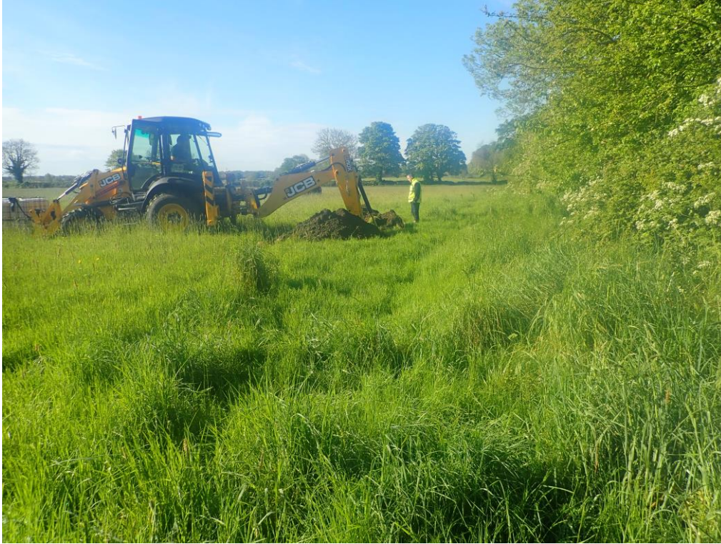
Plate 1: View of the site from the north, while excavating the test holes. See the well drained appearance of the land around the site.
