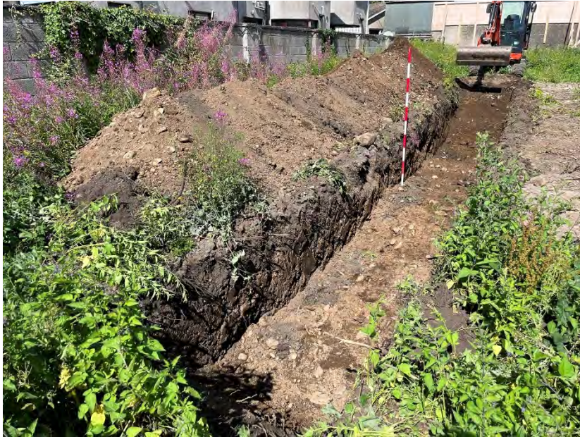
Plate 1: Trench 1 looking northwest
