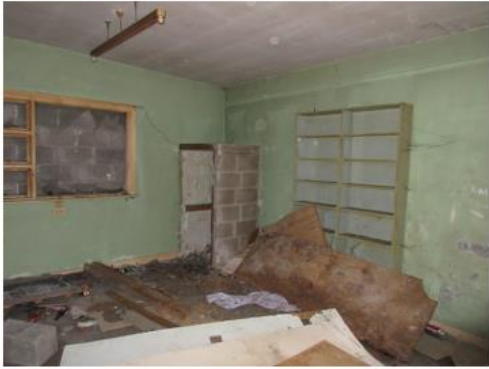
IMG_2926. Interior of Shed 8
