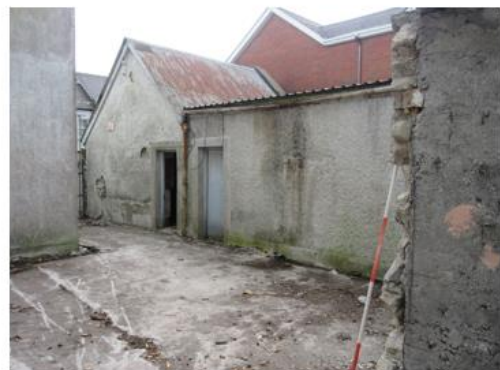
IMG_2933. Building 7. Shed 8 with concrete yard.
