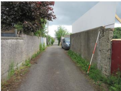
IMG_2952 Back Lane and rear boundary to 43-44 Brews Hill. Facing E
