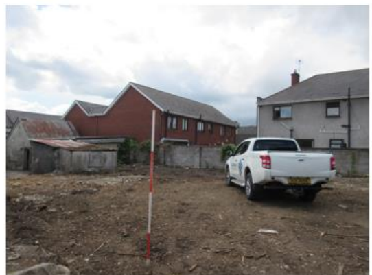
IMG_2917 General from 43 Brews Hill. Facing W
