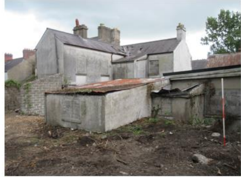
IMG_2935. Rear of Garage 9. with Shed 8 and 43 Brews Hill in rear.
