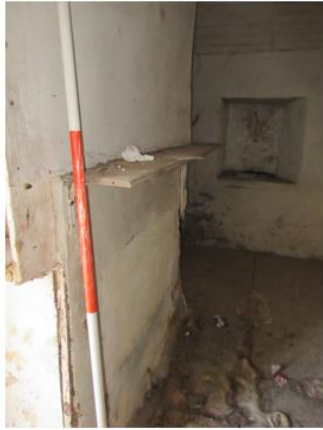
IMG_2918. Building 7. Chimney 7.3 and Window 7.5
