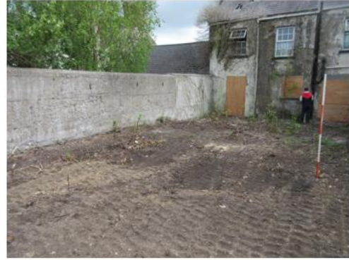
IMG_2943. Concrete boundary wall, concrete apron, Japanese Knotweed and rear of 44 Brews Hill
