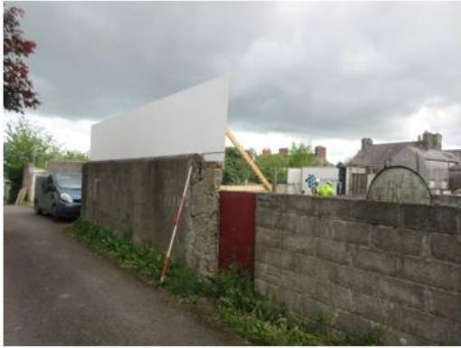
IMG_2950. Back Lane and rear boundary to 43-44 Brews Hill. Facing SE
