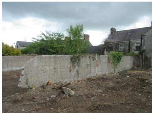
IMG_2938. Mass concrete Boundary 12 between 43 and 44 Brews Hill. Facing SE
