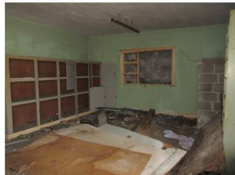
IMG_2925. Interior of Shed 8
