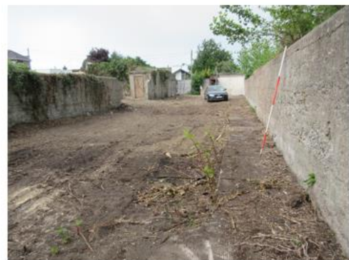
IMG_2949 Rear of 44 Brews Hill Concrete wall and path. Facing N
