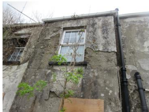
IMG_2947. Mass concrete in rear of 44 Brews Hill
