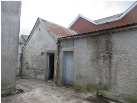
IMG_2922. Building 7 with pitched roof and modern door 7.1. Adjacent Shed 8
