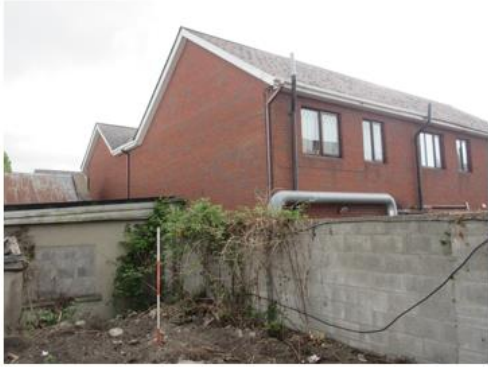
IMG_2934. Left = Shed 8. Right Boundary wall 13
