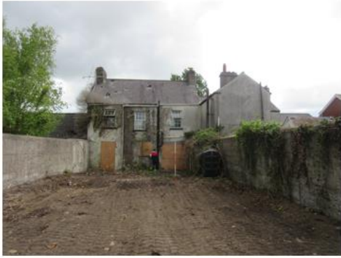
IMG_2942. Rear of 44 Brews Hill. Facing S
