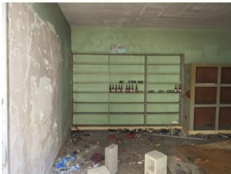
IMG_2924. Interior of Shed 8
