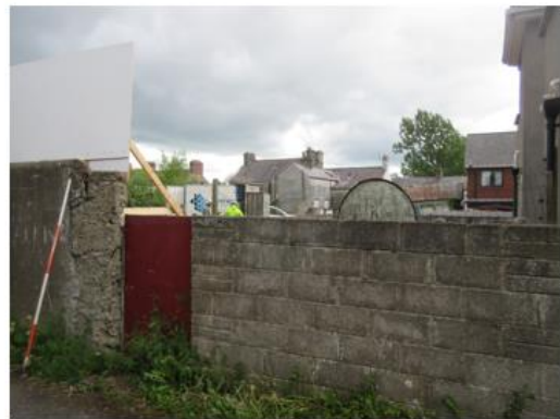
IMG_2951 Back Lane and rear boundary to 43-44 Brews Hill. Facing SE
