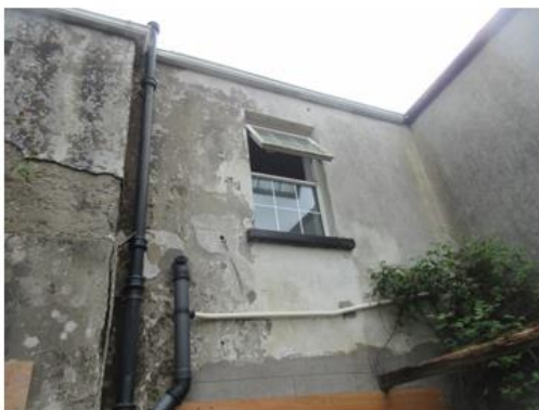
IMG_2948. Mass concrete in rear of 44 Brews Hill
