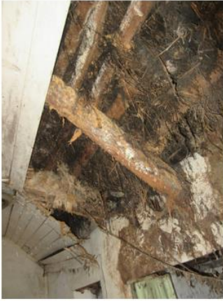
IMG_2920. Roof joists 7.10 with battens and under-thatch
