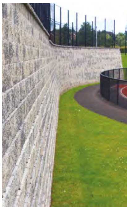
Walling & Retaining Walls
