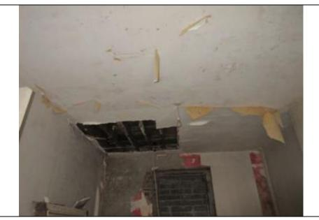
Internal view of No43 with significant damp penetration and collapsed ceilings.
