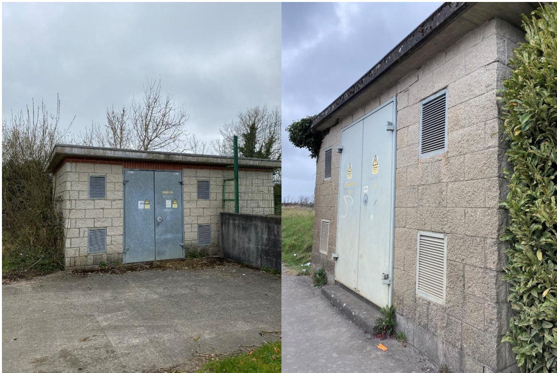
Plate 5.3: Photos showing two electric housing units BL3.
