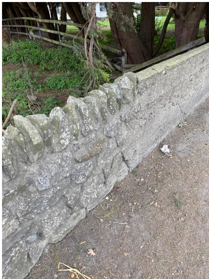
Plate 5.1: Photo showing the stone wall bridge BL1.
