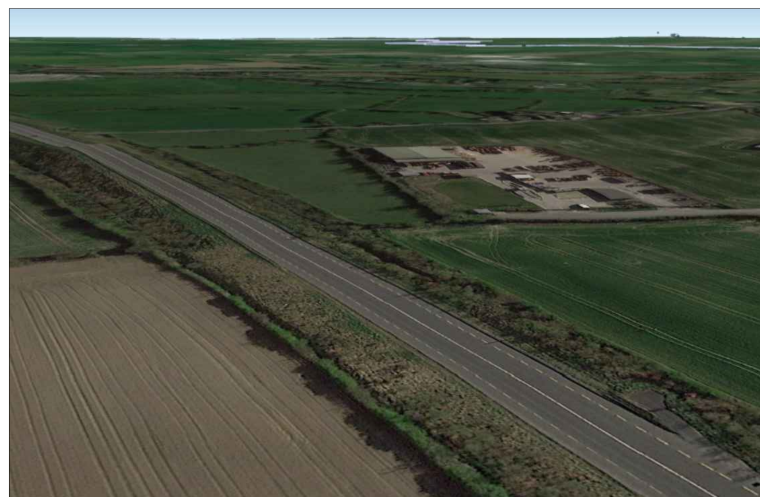
EXISTING R157 VIEW
