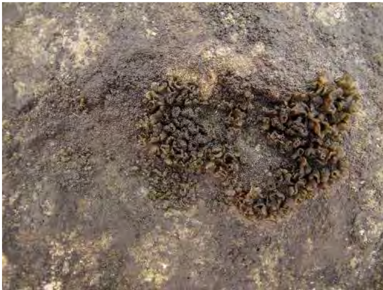
Figure 3: Collema species are rare on the bridge. Again, more of this group should be present if mortar had not been replaced by cement.
