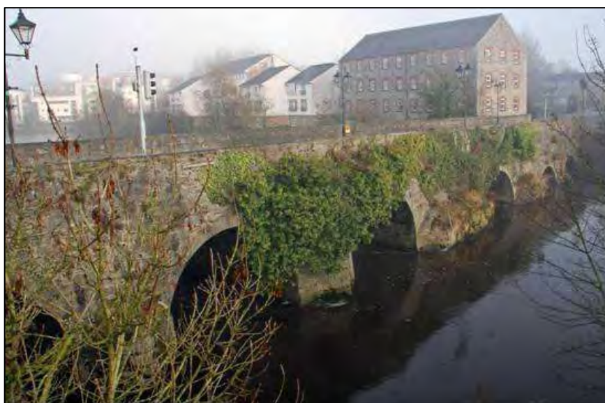
Plate 12: Upstream side of New Bridge, seen from the western bank
