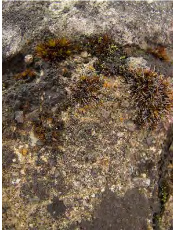
Figure 4: Protobastina rupestris (orange dots) on poor cement pointing.
