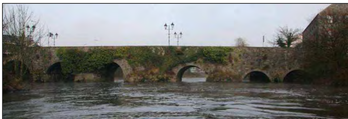
Plate 2: Upstream elevation of bridge (south)
