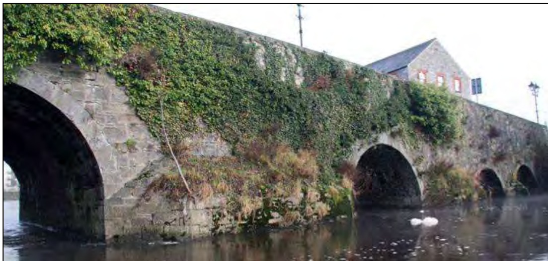
Plate 7: Upstream side of bridge, looking eastwards
