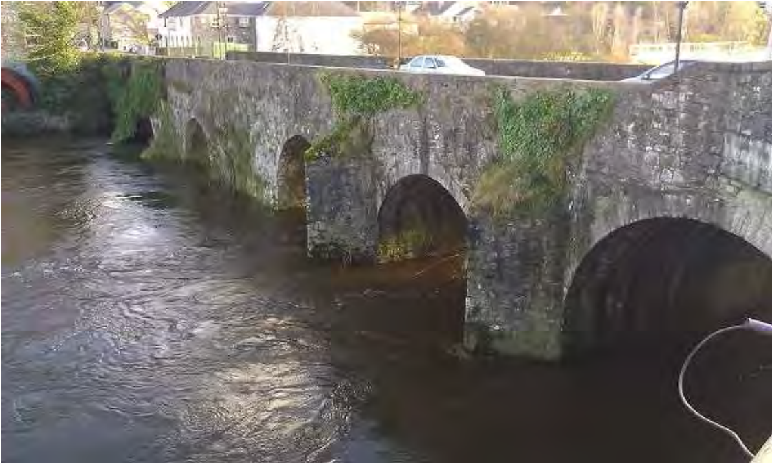
Figure 7: New Bridge, north facing.
