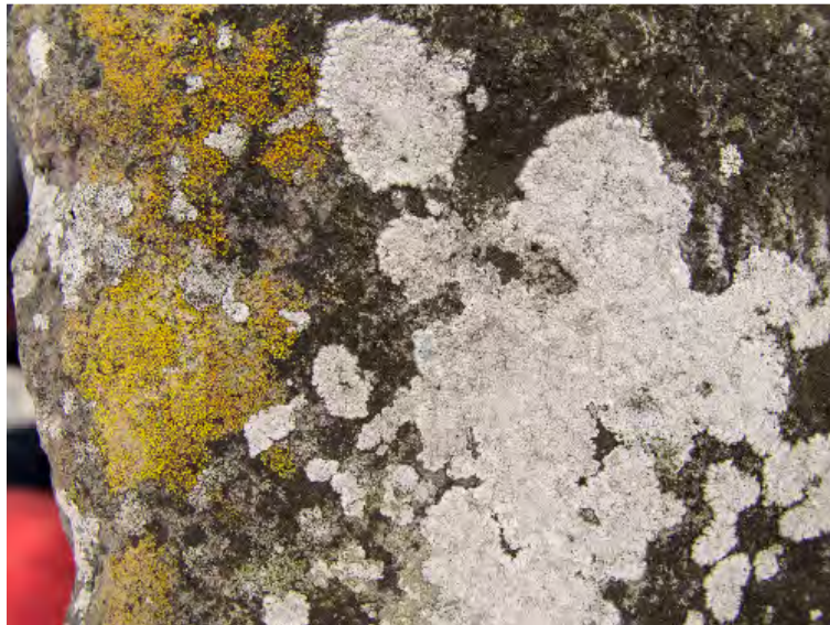
Figure 1: Main species on the bridge limestone blocks are species from the groups Caloplaca (yellow), Verrucaria (brown) and Aspicilia (white).
