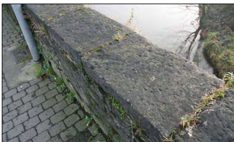
Plate 10: Detail of parapet wall and coping stones
