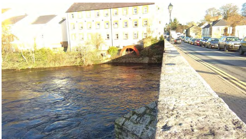
Plate 3: New Bridge with old stone walls (downstream view). Photograph taken in February 2016.
