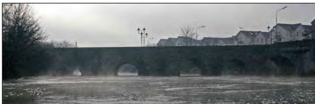
Plate 1: Downstream elevation of bridge (north)
