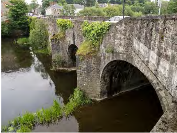
Figure 5: North-facing aspect of the bridge showing large growths of Aspicilia and Verrucaria .
