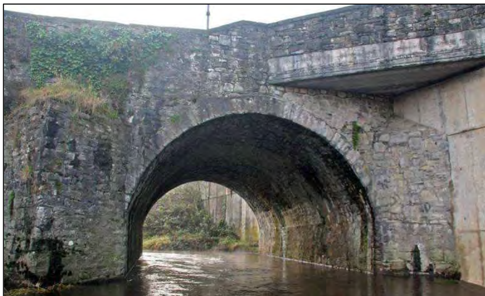
Plate 3: Downstream side of western arch
