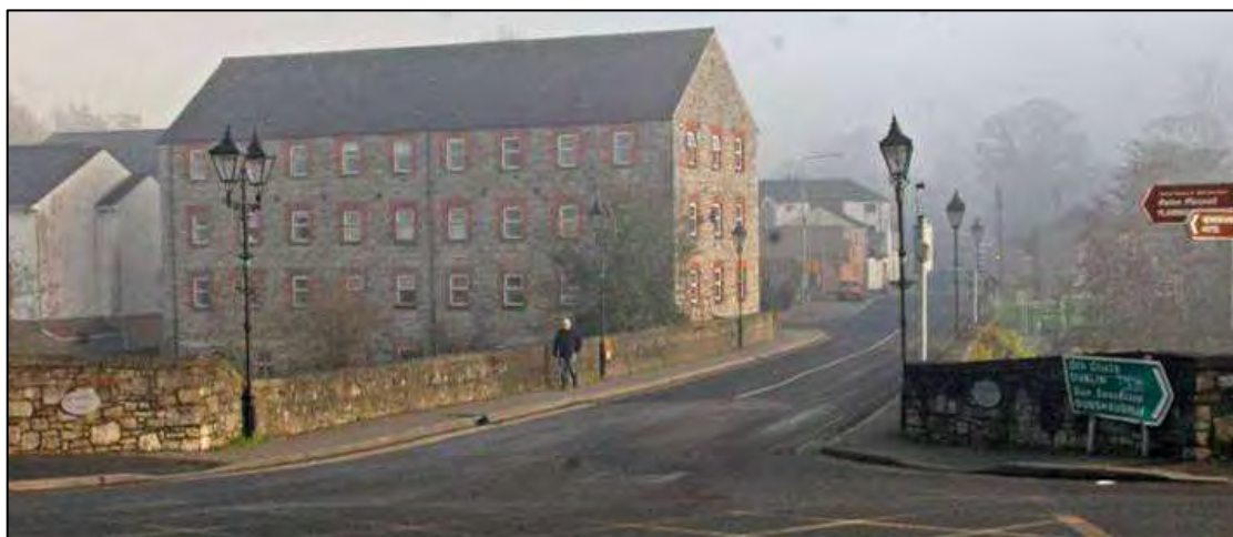
Plate 9: View eastwards across bridge from Navan towards Athlumney
