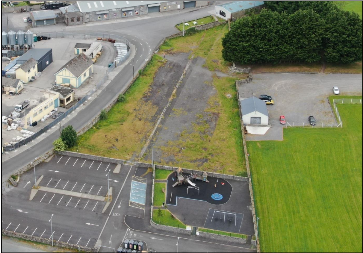
Figure 12: Aerial view of proposed development site
