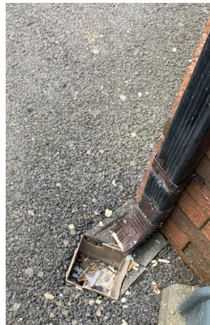
Plate 3-2: Existing drainage channel
