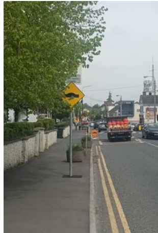
Plate 3-1: Existing Keep Left Sign
