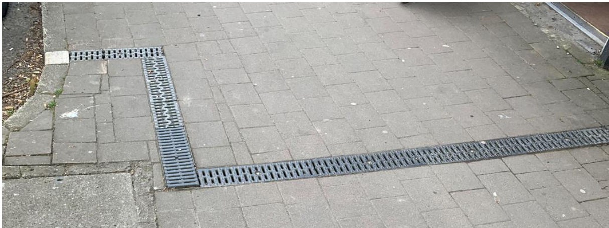
Plate 2-1 Example of existing ACO drain
