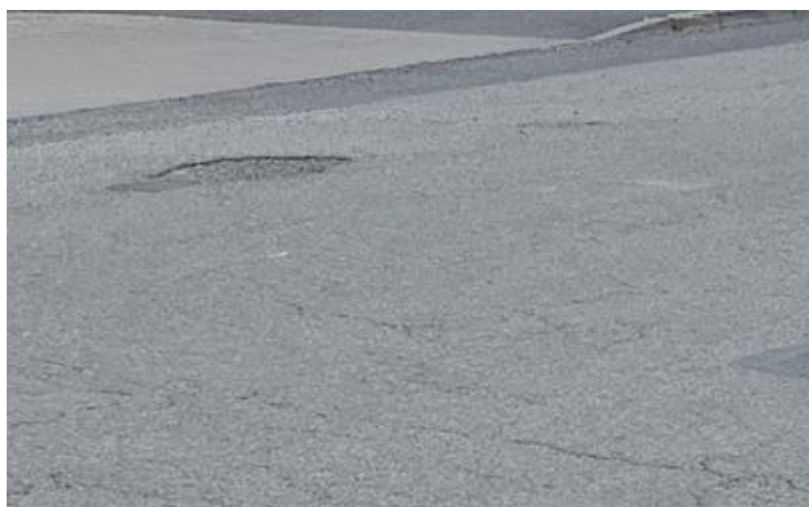
Plate 2-2: Sample of existing access covers.
