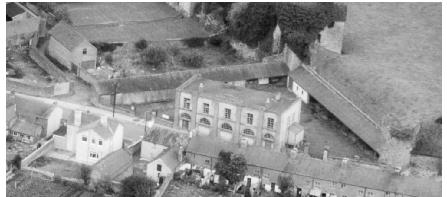
Fig 12. C 1950 General View Trim : Oblique Aerial Photo taken from East - prior to 1950's rear extension being added showing the extent of the 1925 remodelling with market yard to rear.
