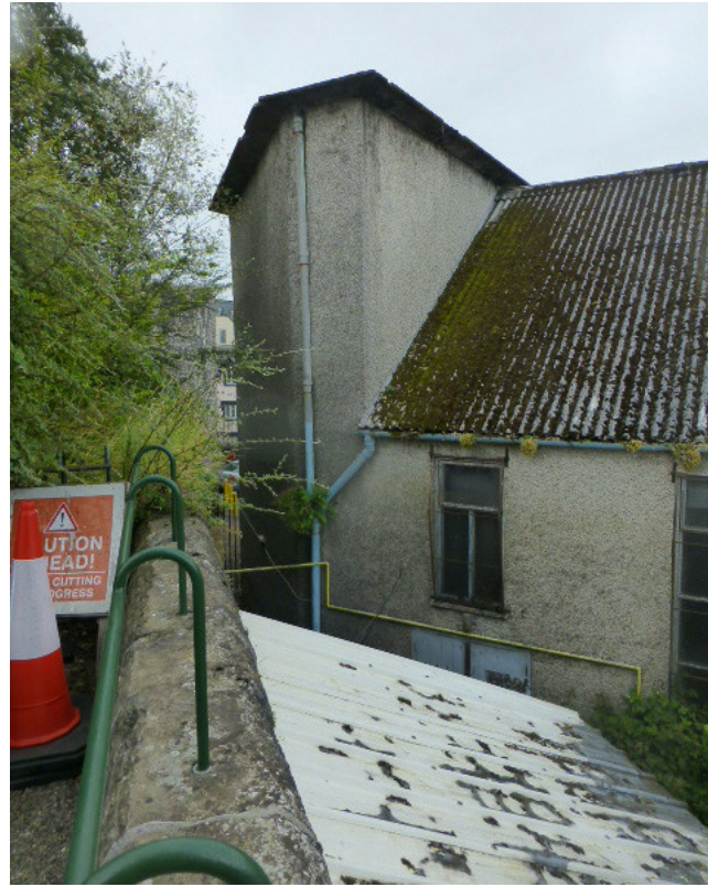
Fig 23. Flat-roofed fly tower terminates south end of the extension .
