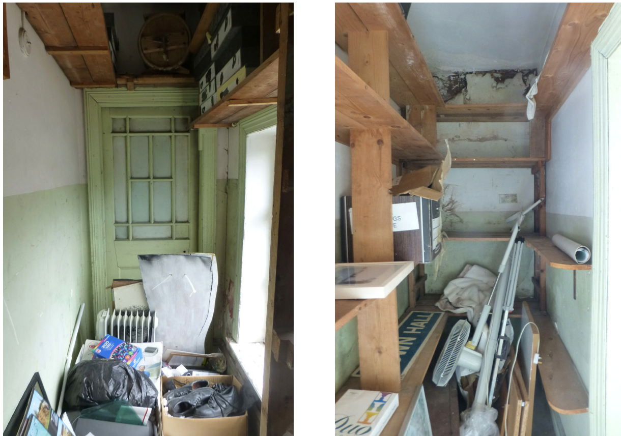
Fig 48.Narrow room with window in side gable
