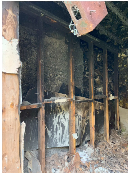
Fig 34. Base of mural tower exposed within lean-to structure.
