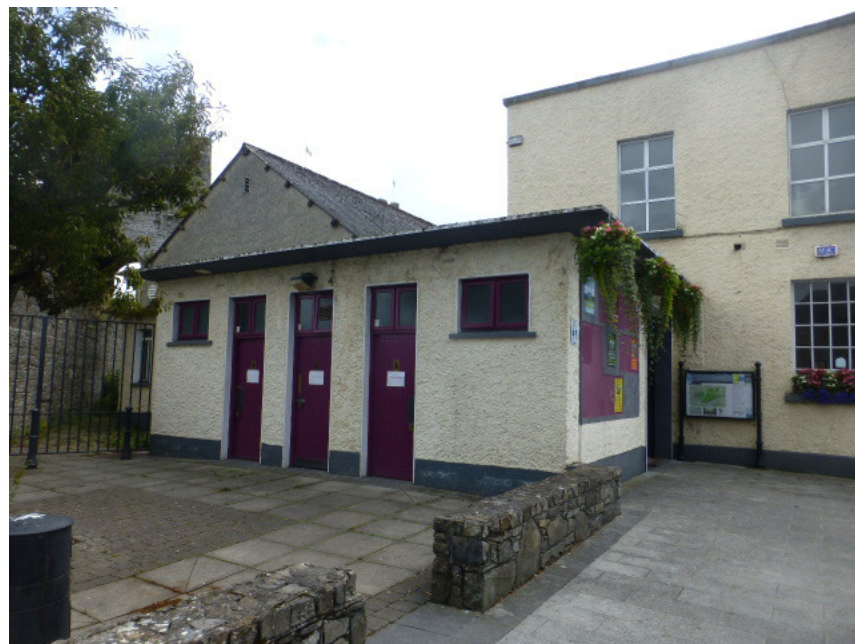
Fig 25. Toilet block - built as part of the 1950's extension.
