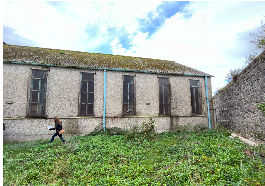
Fig 27. View to rear of 1950's extension.
