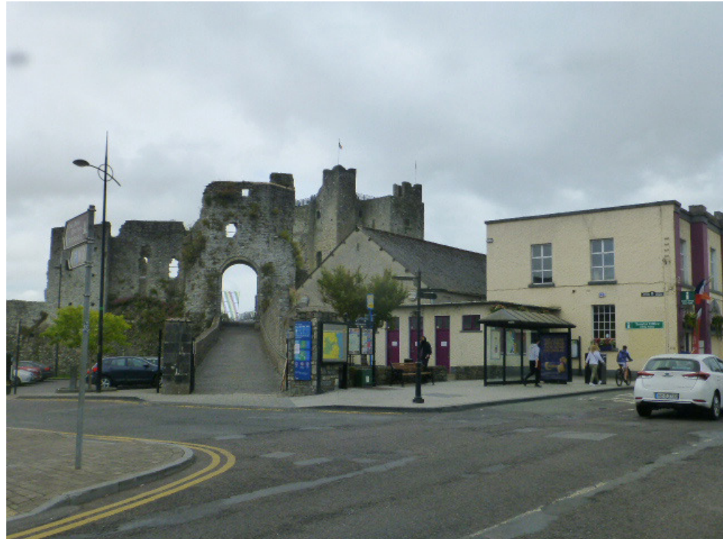
Fig 19. View along Castle Street showing ramped entry to Trim Gate. Flat roofed toilet block extension to north gable of Town Hall/Market House in foreground with ballroom hall to rear.
