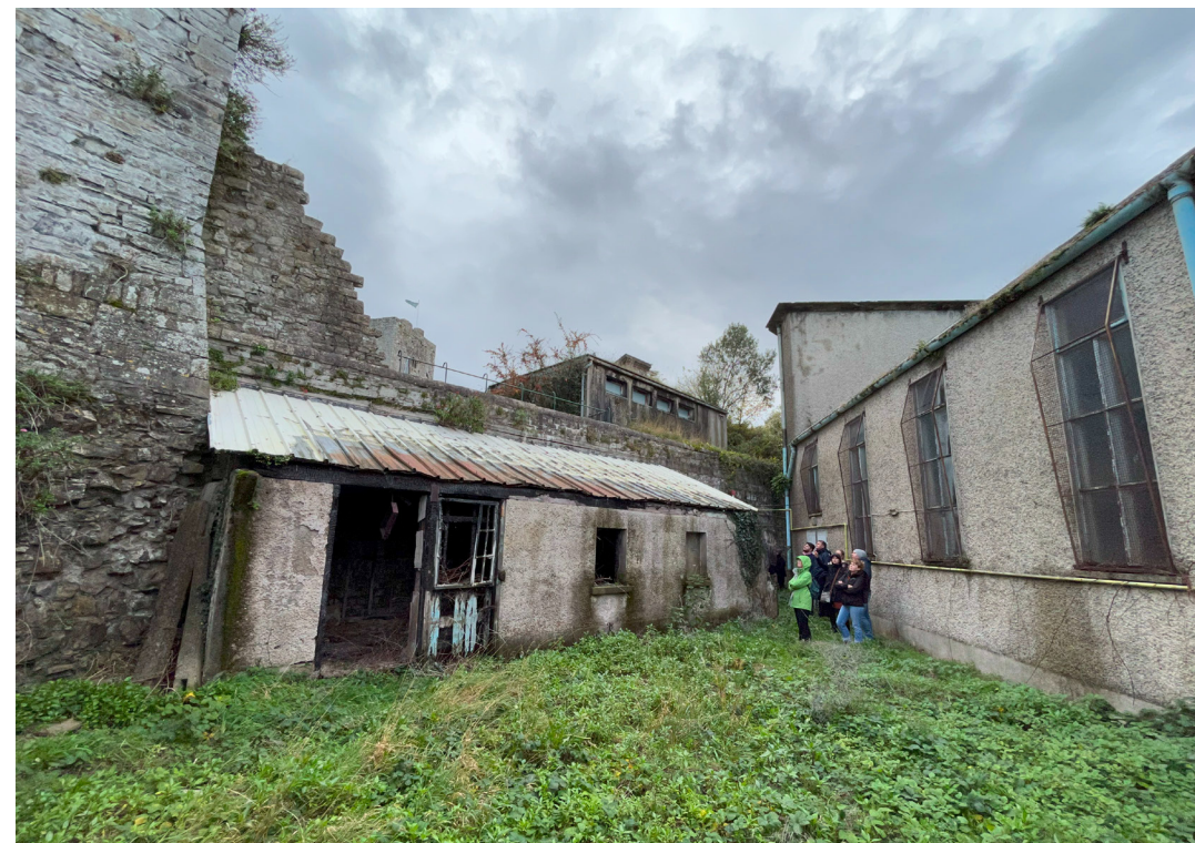
Fig 29. Lean-to structure part of former market yard enclosure.
