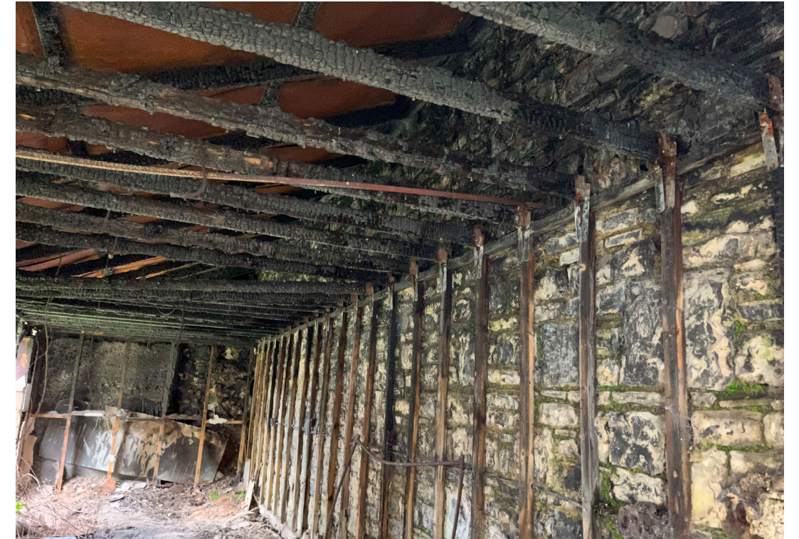
Fig 33. Interior view to Castle curtain wall.
