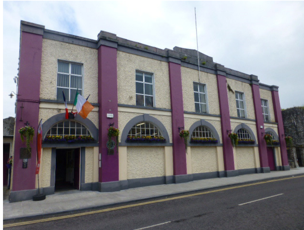
Fig 20. West facing front facade onto Castle Street - advanced three breakfront corresponds to earlier 1850 building.
