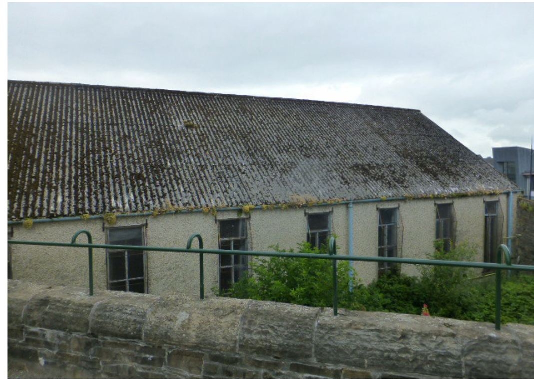
Fig 24. Rough cast rendered 1950's extension with corrugated asbestos sheeted roof.
