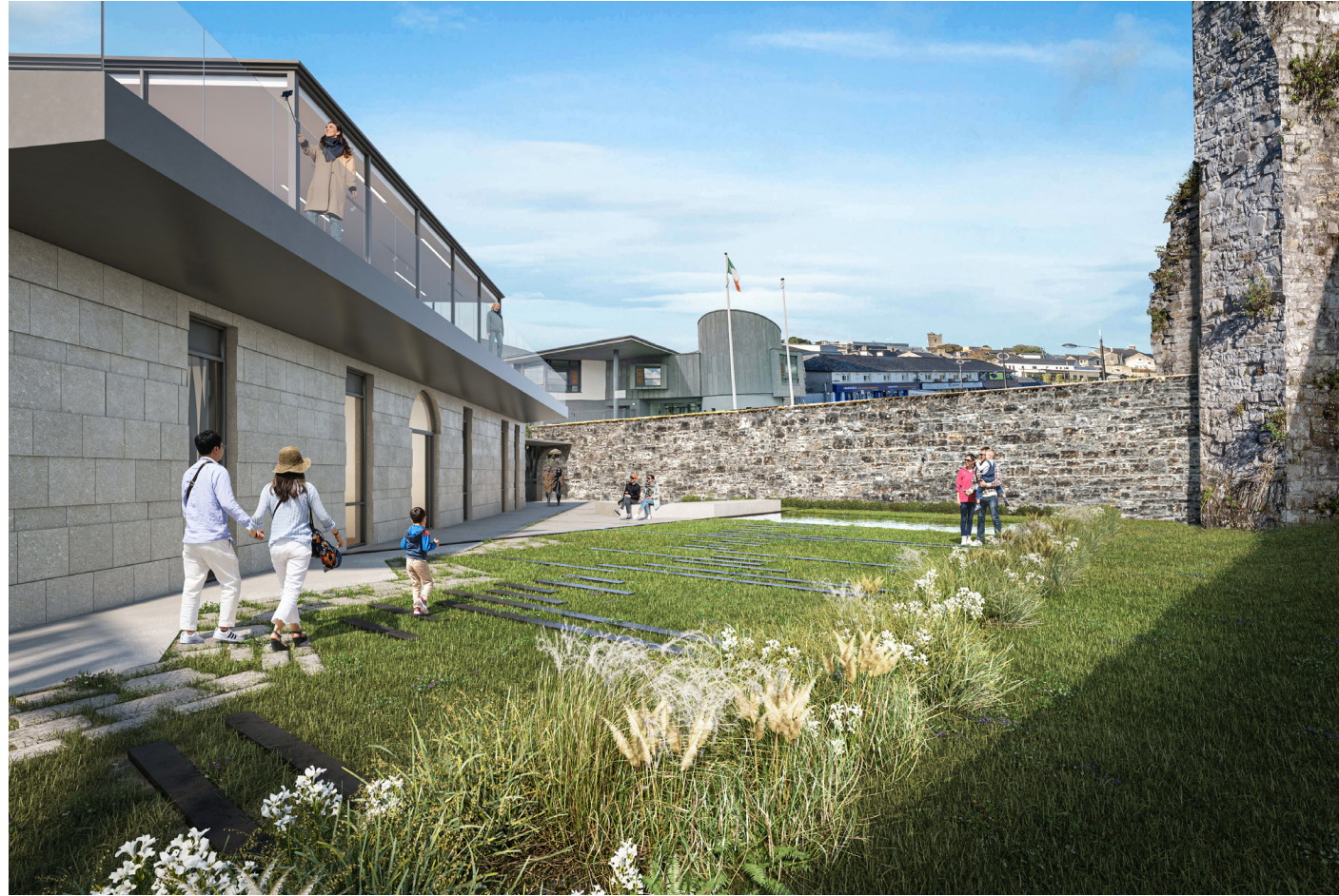
Fig 69. Landscaped spatial separation to Castle curtain walls improves setting.
