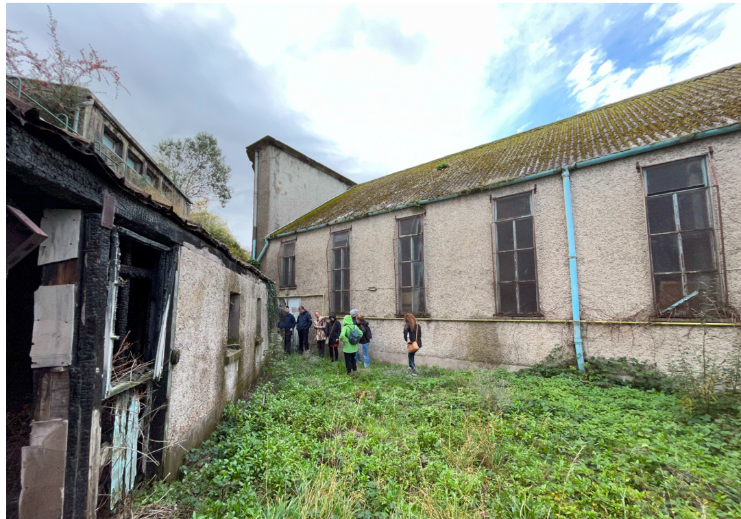
Fig 26. View to rear of 1950's extension.
