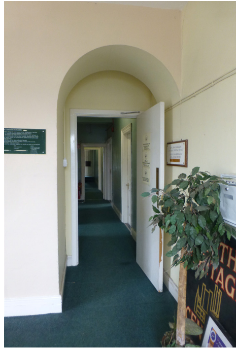
Fig 44. Arched opening formed within former gable of 1850 structure.
