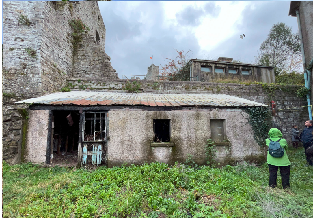
Fig 30. Lean -to outbuilding abutting curtain wall adjacent to Trim gate.
