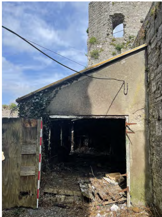
Plate 14: Lean to shed, of modern fabric, along line of structures shown on Du Noyer sketch of 1859 but no evidence for earlier features, burnt inside, facing northeast.
