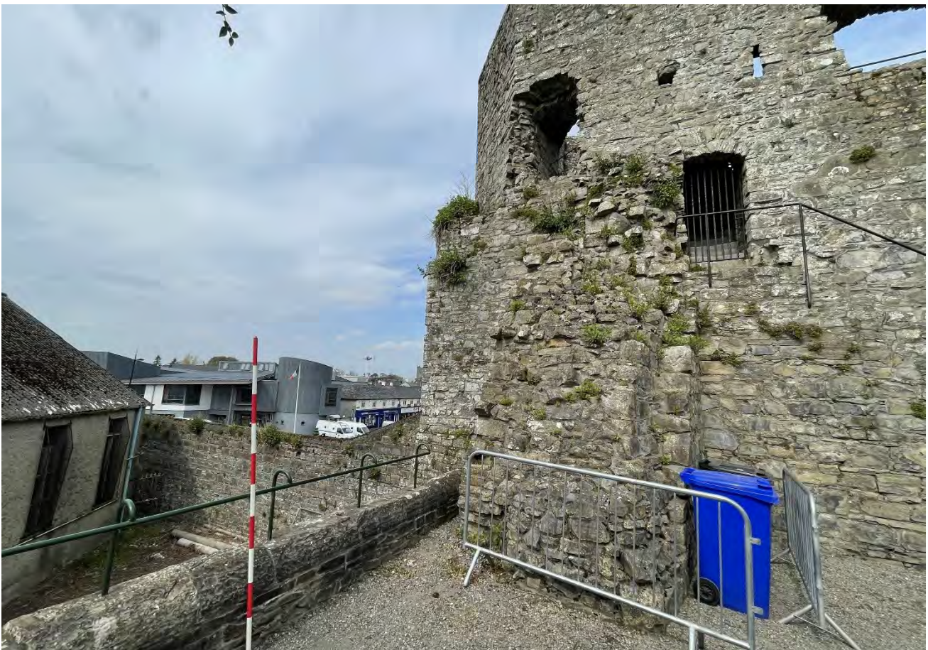
Plate 34: Remains of curtain wall, running off Trim Gate, facing north with modern market wall and rail to left.
