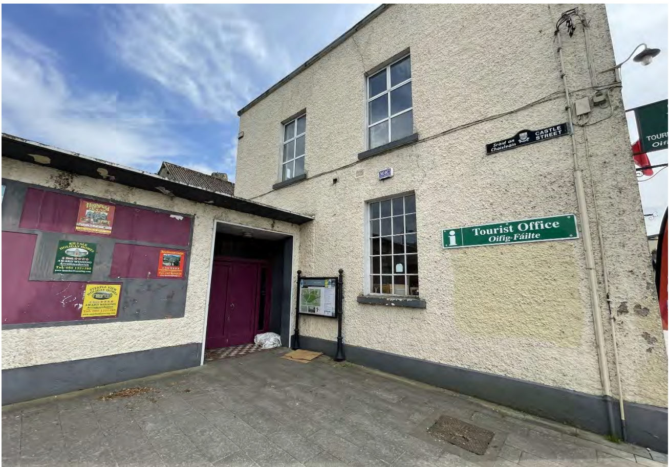
Plate 4: North façade of Market House and extension, facing southeast.
