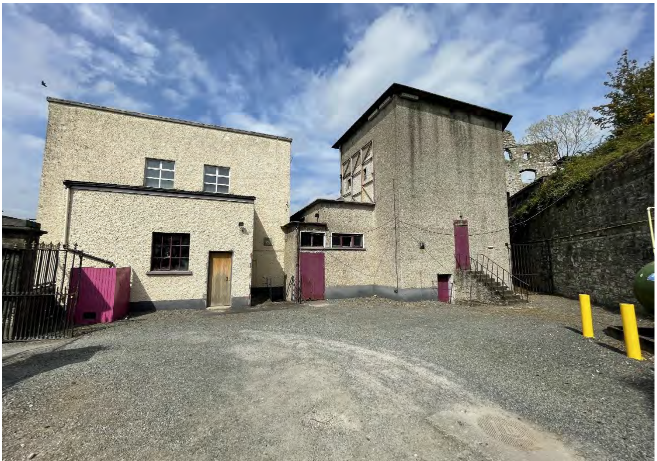
Plate 10: South gable facades of fly-tower of ballroom (to the right) with lean to structure attached to Market House (to the left), facing north.
