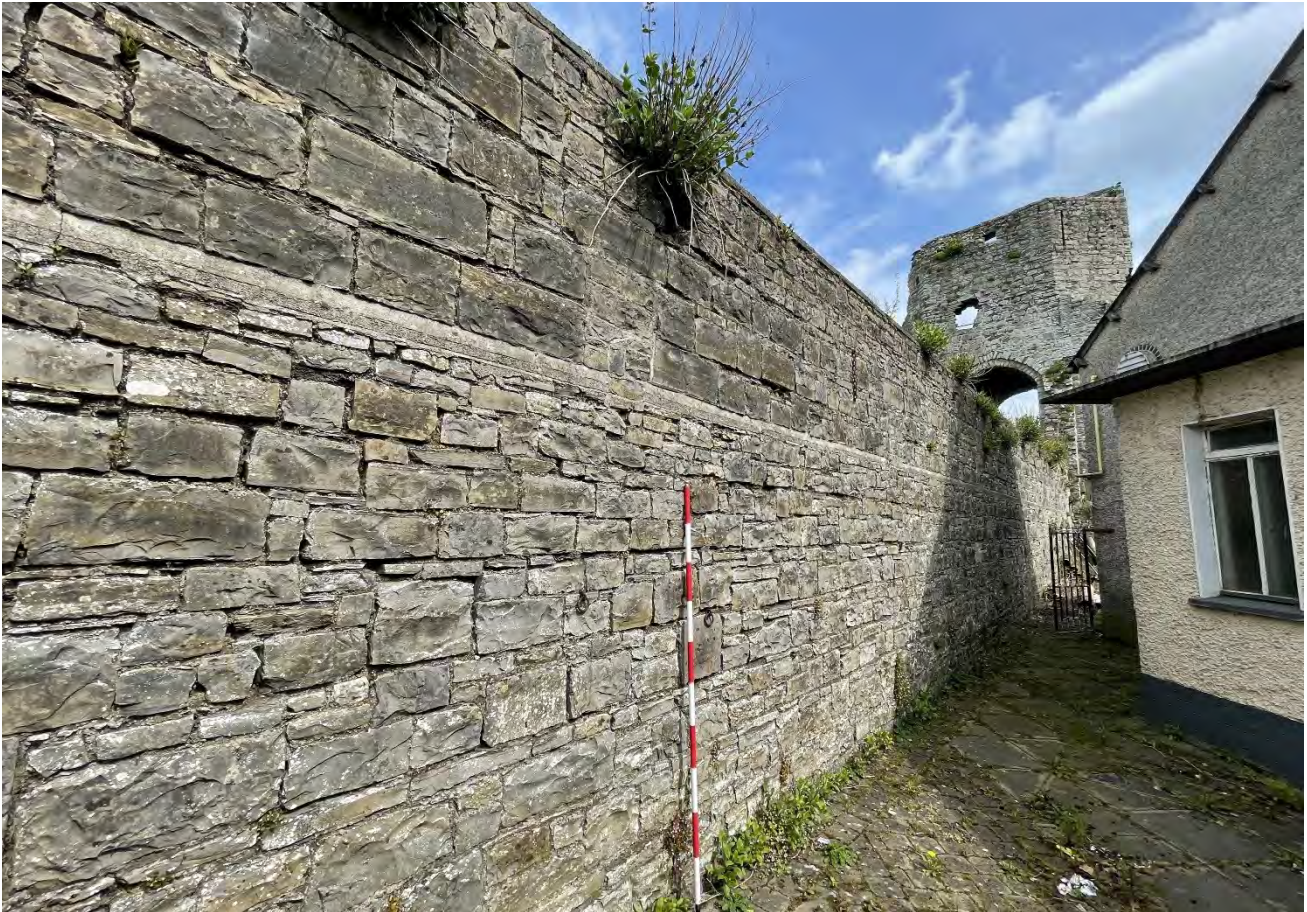
Plate 25: South façade of causeway wall, rear of the site, facing southeast.
