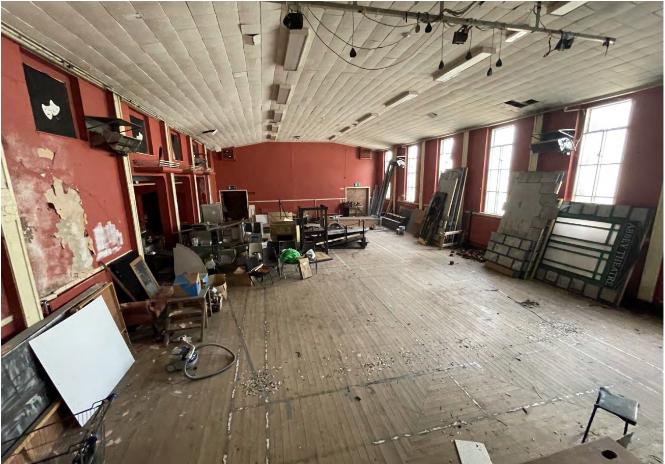
Plate 23: Interior of the Market House Ballroom, facing north.
