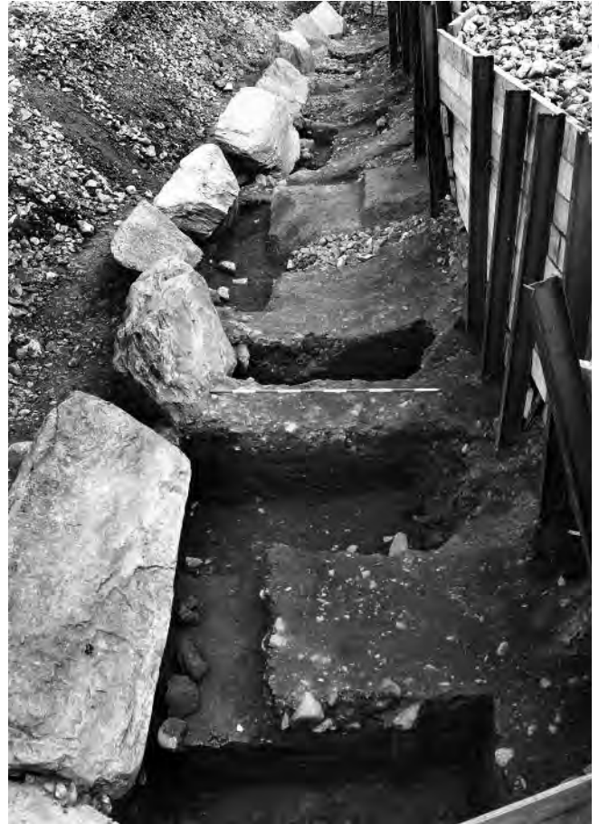
Fig. 13: Excavation of kerbstones and sockets to the rear of the Newgrange tumulus
