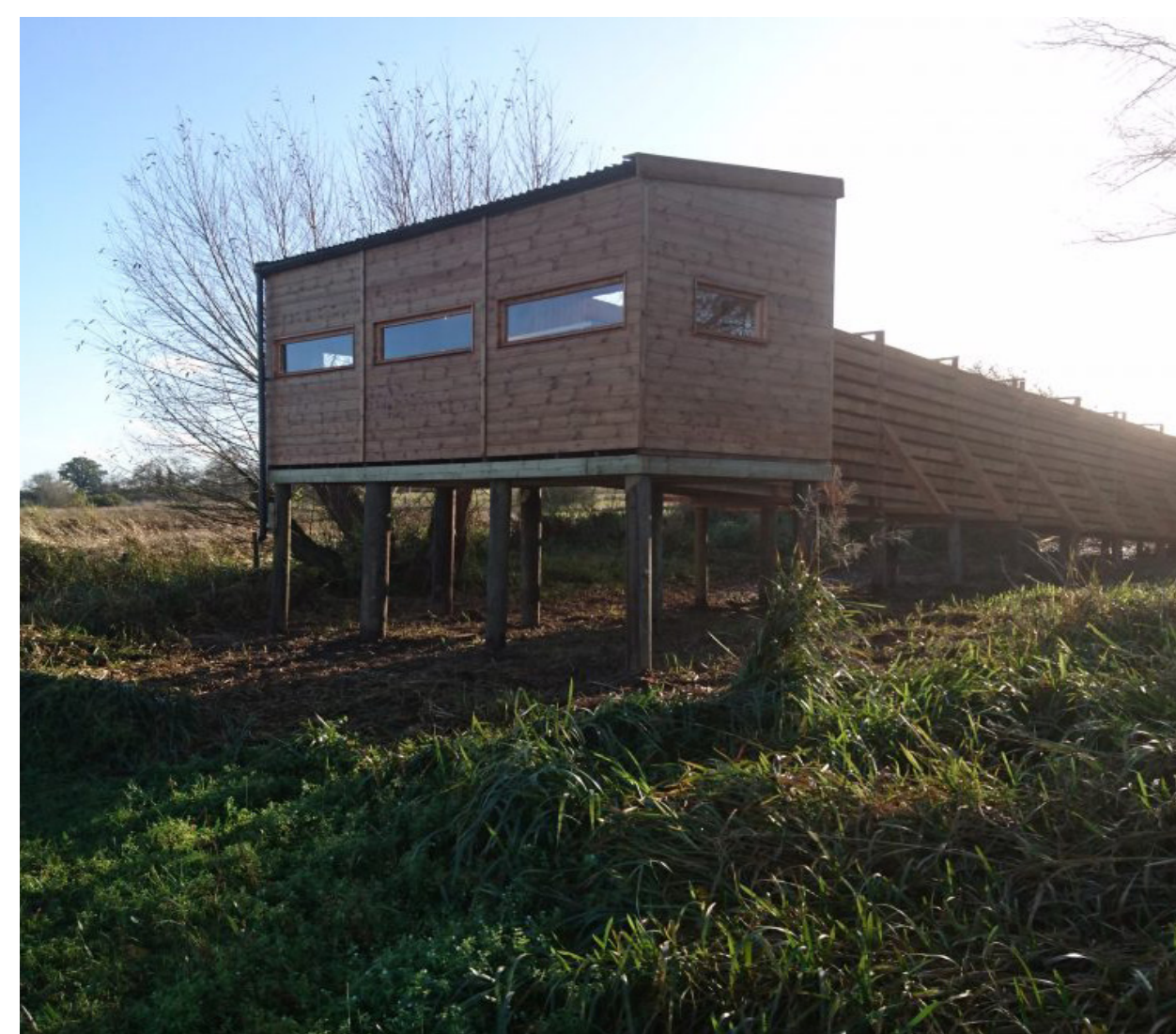
Bird hide composed of timber materials with glazed hatches and rear universal access ramp with a high degree of light and shadow reduction.
