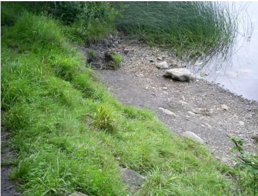
Figure 6: Severe erosion around informal angling stand
